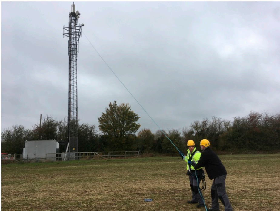
Figure 3. Picture of pull application on lattice towers during modal test.
