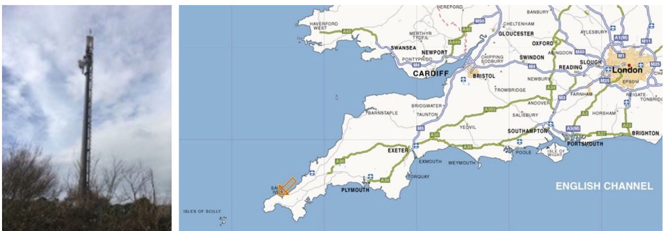
Fig. 1 (Left) Picture of St Ives FC Portasilo monopole. SHM system install. Arqiva. (Right) Location of St Ives in South-West of the UK
