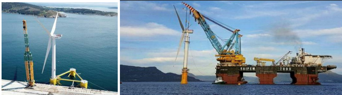
Figure 6 Fit out of semi-submersible, ref [11], and Spar ref [8]
