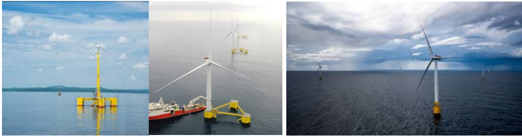
Figure 8 Semi submersibles operating, Ref [13], Ref [11] and Spar operating Ref [8]
