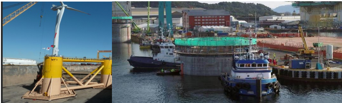
Figure 3 Loadout of steel semi-submersible, ref [11], and concrete Spar ref [8]
