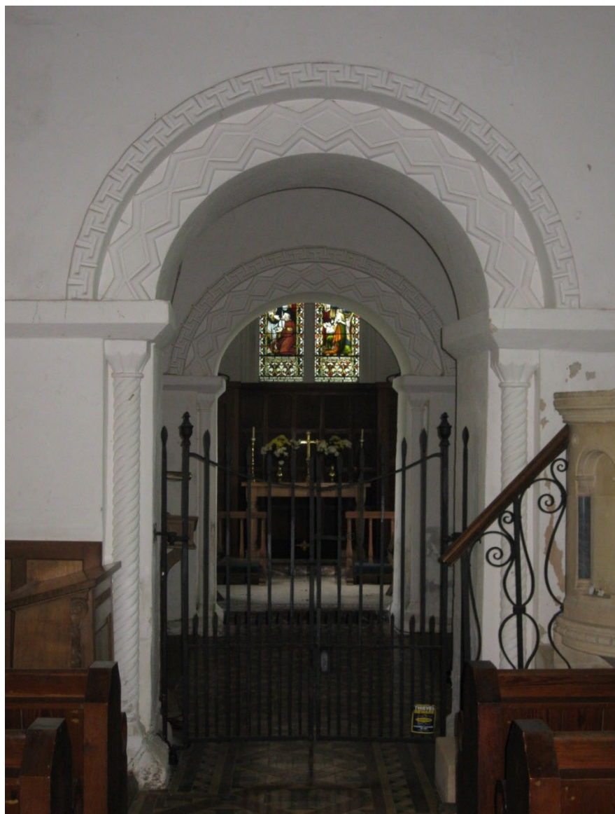
Figure 4.4. The church of the Blessed Virgin Mary [modern dedication], Christon: an apparently fine example of two early medieval or early Norman arches either side of a central tower, but all is not as it seems as they were heavily restored using plaster in 1875 (author's photo).
