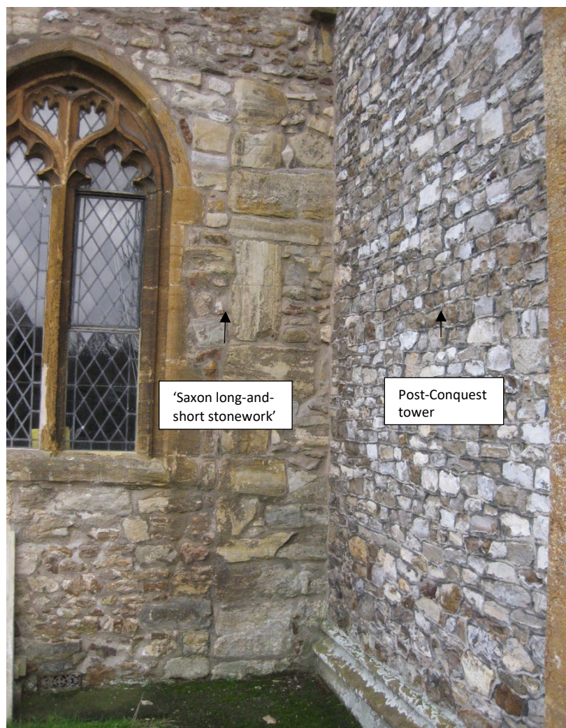
Figure 4.2. St George's church, Wilton, showing extant 'Saxon long-and-short' stonework in the west wall, the tower is to the right (author's photo).
