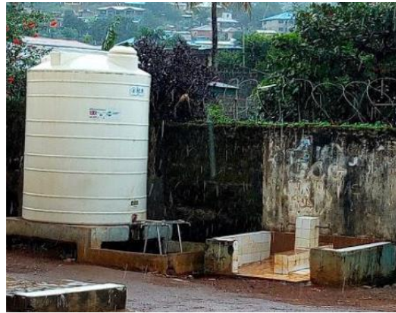
Figure 5. 1 A 10,000 L tank located next to a public standpipe point at Wellington
