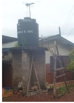
A private installed water tank at Kissy
