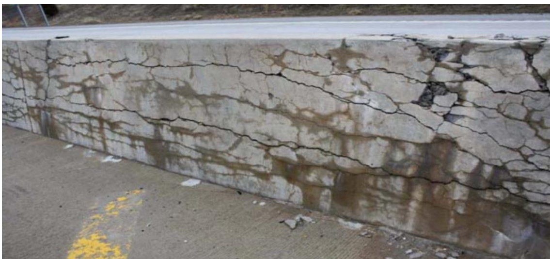
493 Figure 4: A highway barrier deformed by alkali-silica reaction (ASR) (Akhnoukh 2013).
