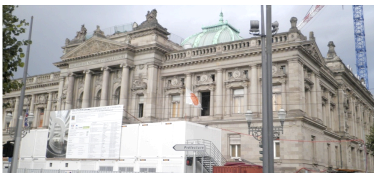
8. The Library undergoing renovations on 09/08/11. © Isaure Triby
