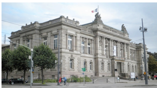
7. The permanent building for the Delegation, now housing Strasbourg's TNS, on the 09/08/11. © Isaure Triby
