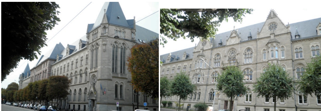
9. Two views of the Gothic Central Post Office’s fronts from opposite sides. The photo on the left shows the main entrance’s side (09/08/11). © Isaure Tribay
