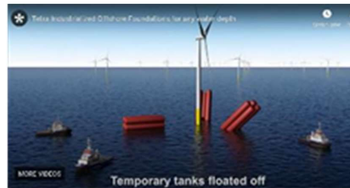
Remove temporary buoyancy after Connecting tendons
