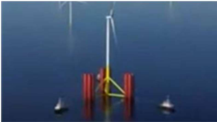
Tow out with temporary buoyancy
