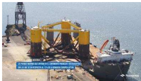
Figure 7 Semi submersible loadout onto HTV(Principlepower website, 2022)
