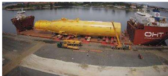
Figure 8 Spar loadout onto HTV (Equinor website, 2022)
