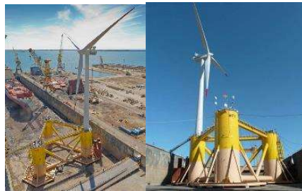
Figure 6 Semi submersible constructed in dry dock, (Principlepower website, 2022)
