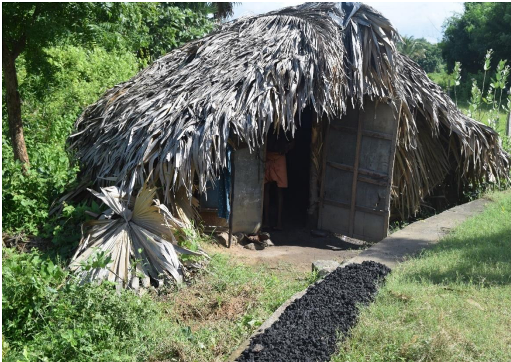
Figure 5.10 Typical forge hut made from palm fronds in Kollengode. Note charcoal drying in the sun.
