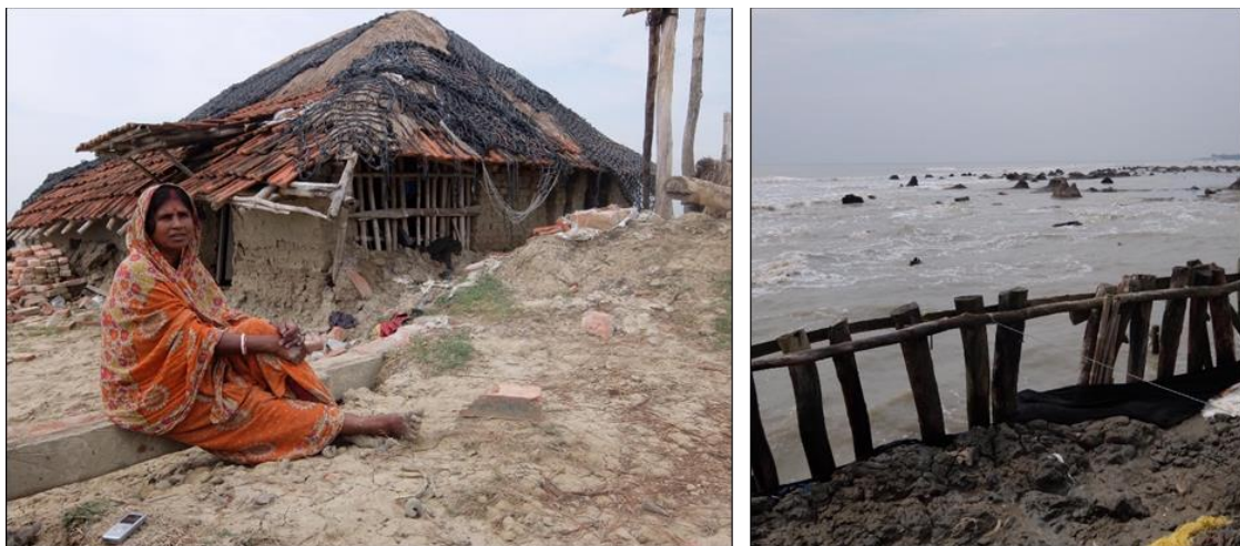
Image 3.5. Dwelling on the coastal area of Dhablat that has been damaged by floods and recurrent storms (left) and the coastal embankment in Dhablat (right).
