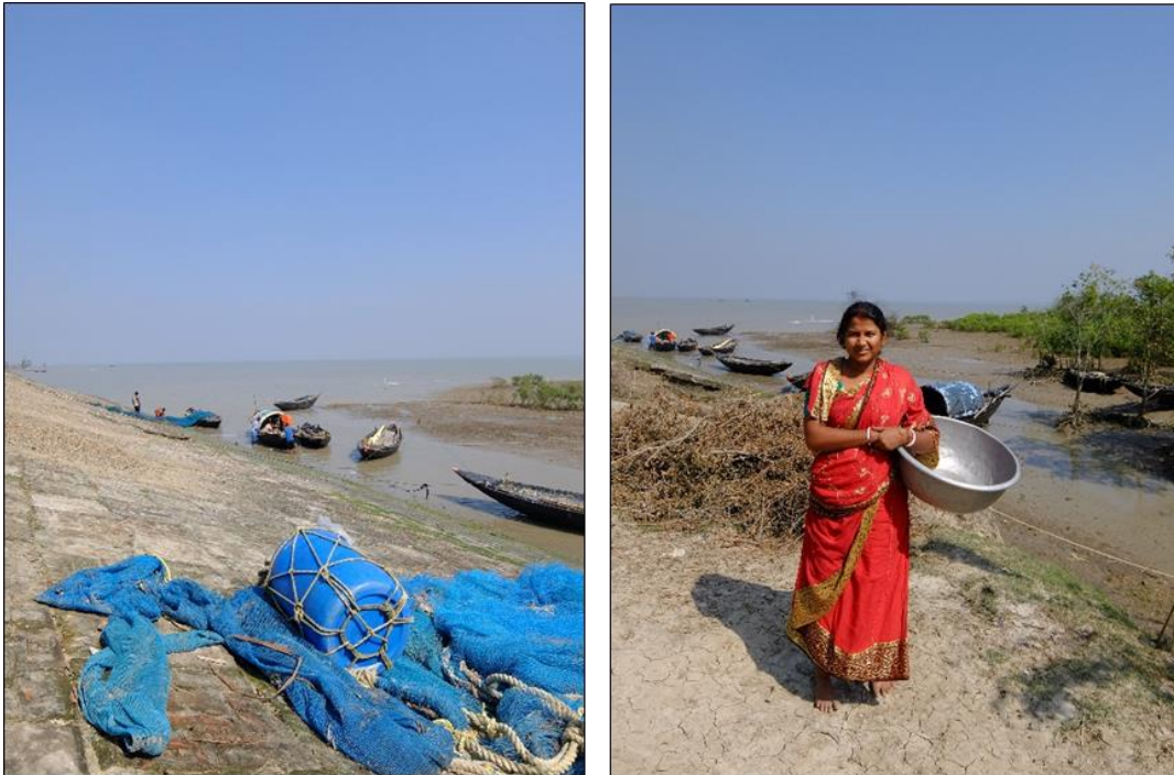
Image 3.4. The embankment in Beguakhali (left) and the area between Beguakhali and Dhablat where the embankment ends (right).
