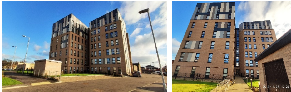
Figure 1: Two views of the Yoker building.
