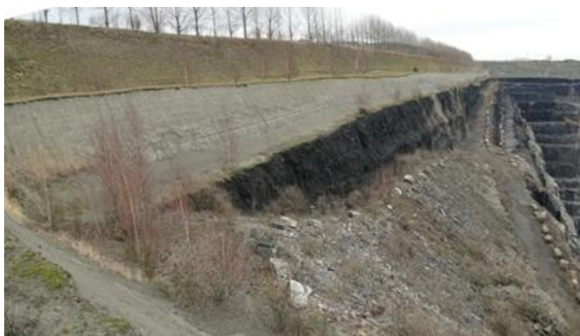
Figure 4. Layers of grey silty sand forming the overburden at a large open pit quarry for limestone; a layer of dark limestone is visible in between the burden and rock benches (credits C. Oggeri).
