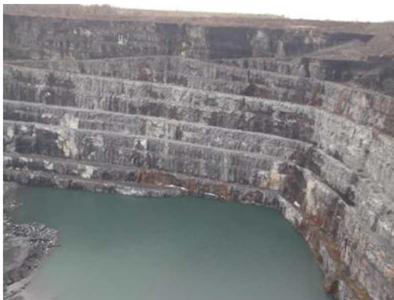
Figure 1. Open pit lake, with raising water level in the basin, ready for backfilling (credits C. Oggeri).
