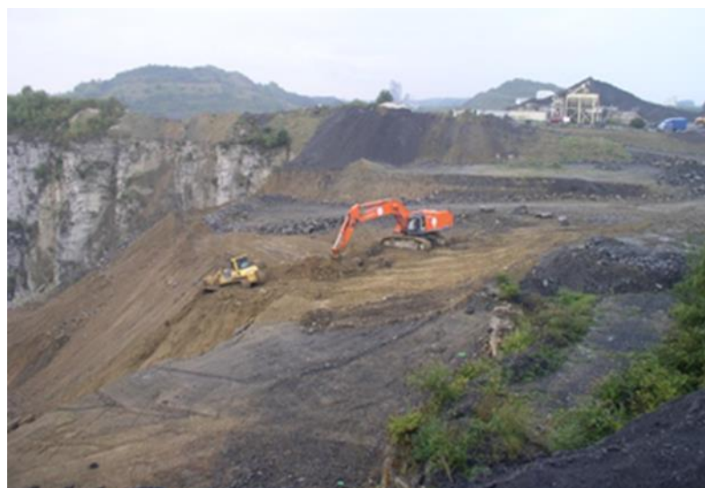
Figure 2. Burden disposal by direct dumping in exhausted open pit (credits C. Oggeri).
