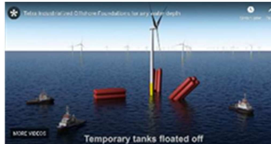
Remove temporary buoyancy after Connecting tendons
