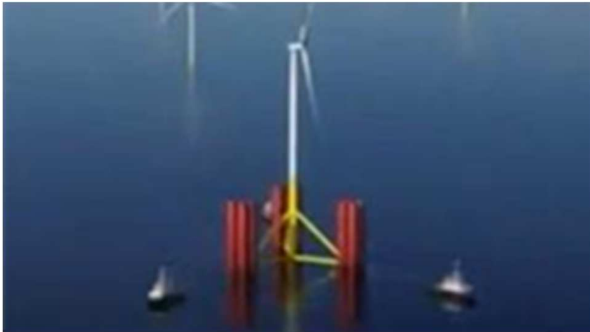
Tow out with temporary buoyancy
