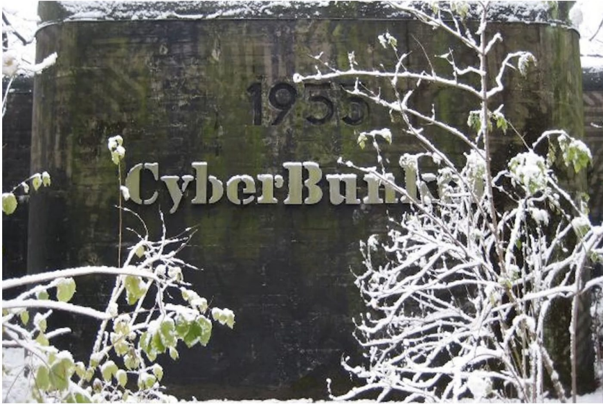
Figure 7. The CyberBunker data centre promised its clients ‘bulletproof web hosting’. It was known for hosting phishing sites and other websites linked to the dark web (Caesar, 2020). Despite its ‘bulletproof’ exterior, in 2002, the servers were removed from the facility after a fire broke out, revealing that the site had also hosted an MDMA manufacturing lab (image reproduced under Fair Use Licence).
