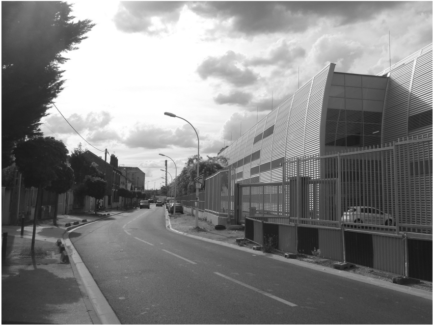
Fig. 4.1: Interxion Data Centre Par7 facing the houses of the rue Rateau. Photo by author.
