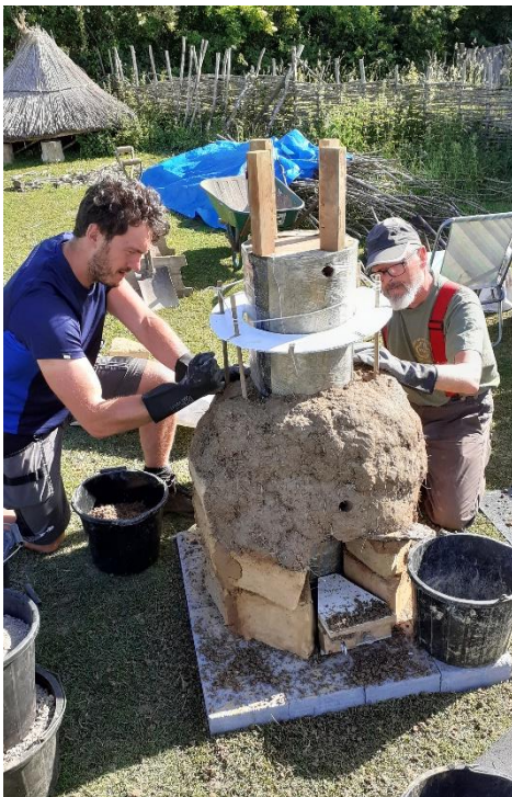
Figure 4.74 - Building a furnace at Cranbourne by daubing clay (the furnace lining) around a forming mould. The clay in this instance was tempered with straw and sand, but tempers can also include small stones (Dungworth et al 2012) and crushed furnace linings from earlier furnace structures. (Author's image).
