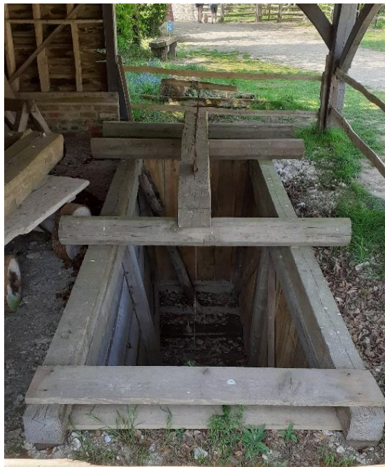
Figure 6.27 (right) – Reconstructed sawpit. This example was covered by a timber framed building suggesting longevity of use. It is unclear how long the sawpits remained in use for at Tudeley. They may have been reused over successive seasons or dug temporarily to process timber felled from an adjacent tree. (Author's image).
