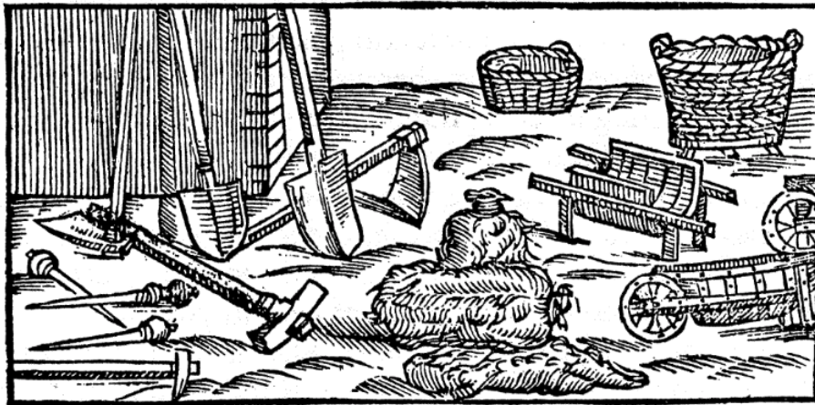
Figure 6.33 – Biringuccio's 1540 illustration of 'Miners' tools, ore barrows, and baskets'. Biringuccio says '...powerful tools are required, like large hammers and iron picks, long thick crowbars, mattocks and strong spades, picks both with and without handles, and similar iron tools, all of fine and well-tempered steel...' (Mudd 1942, 24). The Tudeley accounts record various tools used by the works to process the ore which included 'two troughs bought to carry stones' and 'a hand cart' bought in 1350-51 and a 'hammer for breaking stones' in 1354. Image courtesy of Mudd (1942, 24).
