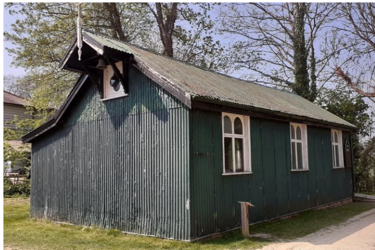
Figure 4.58 – The Tin Tabernacle from South Wonston, Hampshire shows how the ‘iron church’ at Roffey would have once appeared (see figure 4.59). Author’s image.
