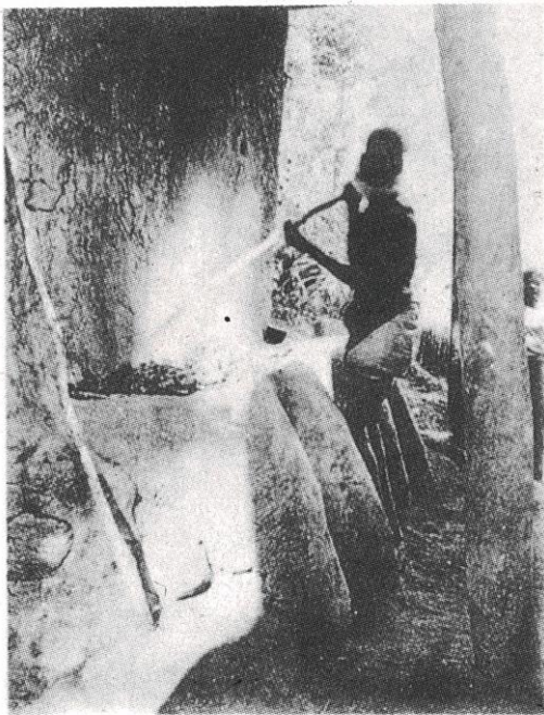
Figure 5.68 - Use of a boring stick, photographed by the wife of Ananda Coomaraswamy in c.1908 in a village ironworks in Sri Lanka. The significance of the boring stick in this photograph was recognised by Juleff (1998) as one of the boring sticks referenced in the song ‘Treading the Bellows’. Image courtesy of Coomaraswamy (1956) plate LIII.
