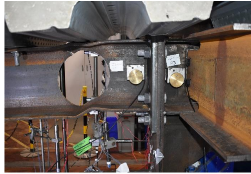
Top crack at the end of first cycle of 0.05 rad (hogging).
