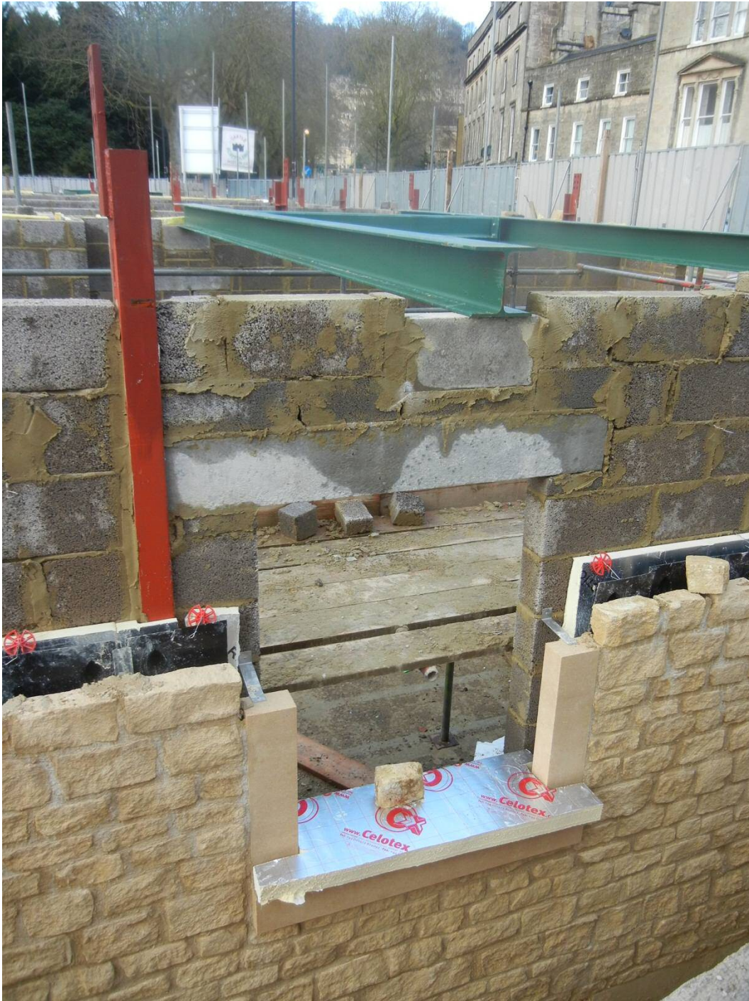
Figure 2.2 - Detail of a cavity wall construction with a concrete block inner face and a stone outer face with intermediate insulation.
