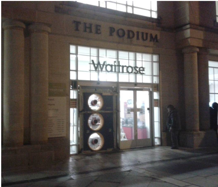
Figure 2.3 - Three fans installed in one of the entrances of a recently refurbished supermarket to test its air-tightness. Bath, November 2012.
