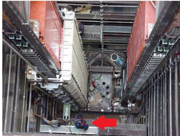
Figure 30 Direct drive PMLG in AWS compared with human size (Polinder, Mueller et al. 2007)
