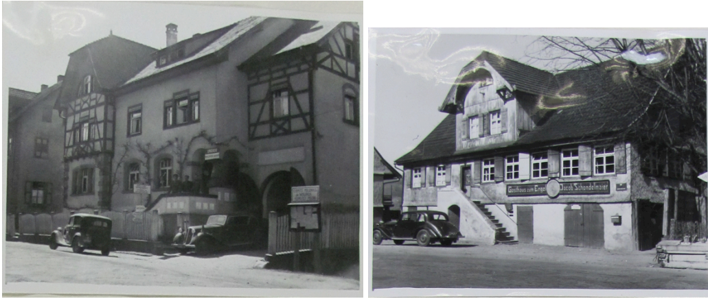
Fig.20/21/22/23. UNRRA buildings under the direction of UNRRA Team 572, Gutach area. 114
