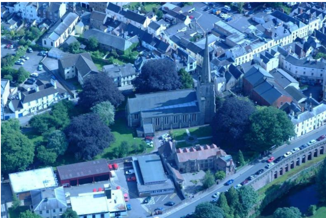
Fig.7.10. Aerial view of St Mary's, Monmouth (© Crown Copyright - Royal Commission on the Ancient and Historical Monuments of Wales).
