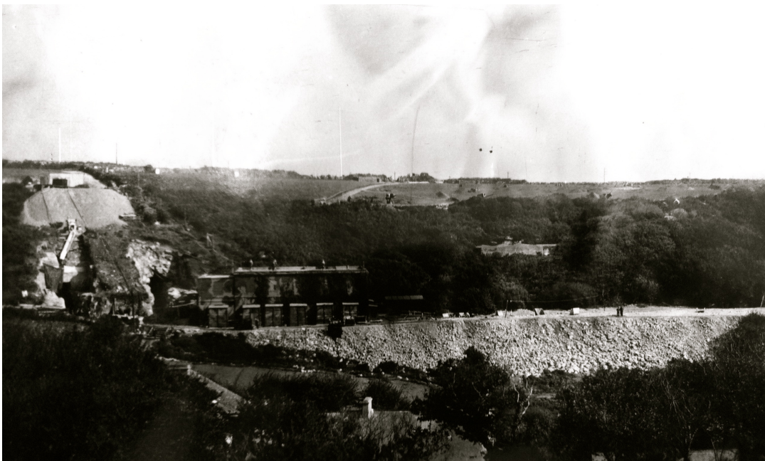
Figure 7 View of Instrument Room: tunnel construction to the left of the frame; spoil tip extending across to the right
