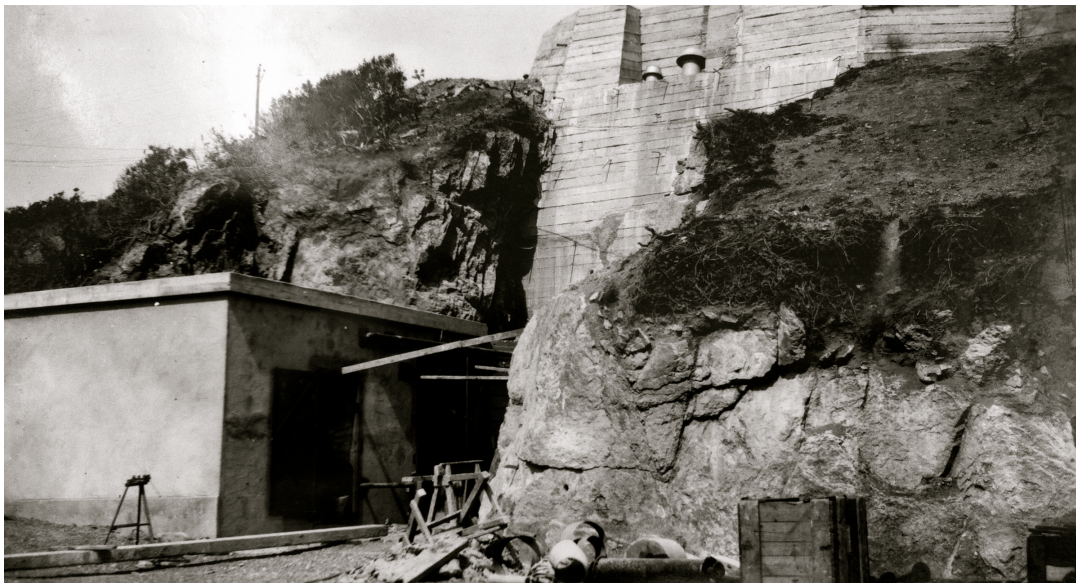
Figure 9 Entrance to Tunnel 2 - the engine room and plant.
