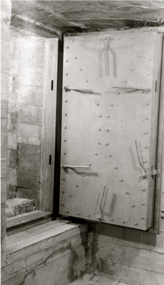
Figure 12 Gas, blast and Commando proof door at entrance to tunnels.
