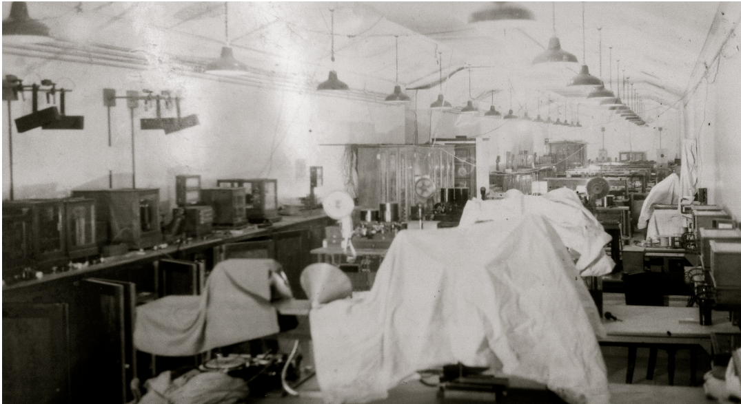
Figure 10 View of newly completed Instrument Room (Tunnel 1).
