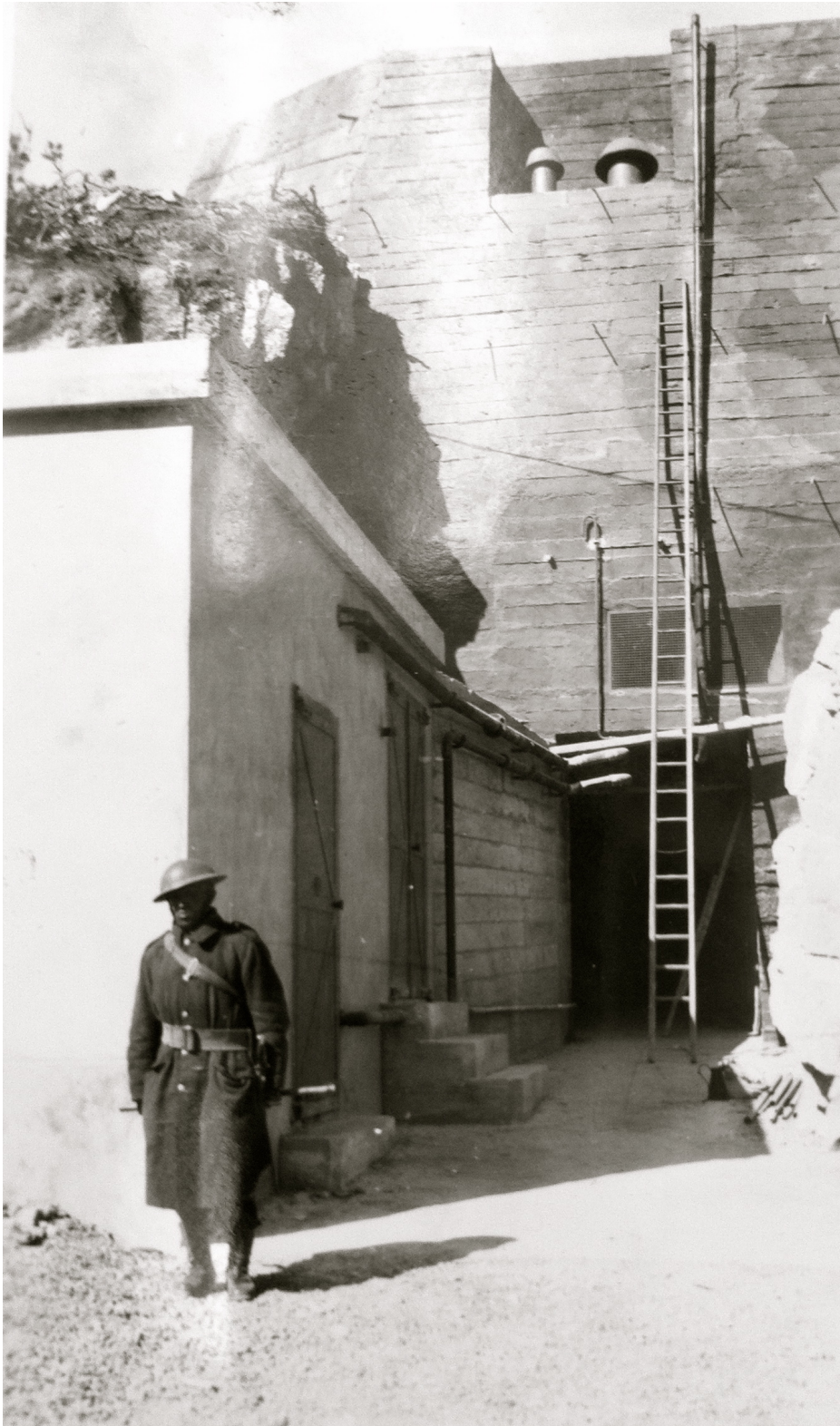
Figure 11 Entrance to Tunnel 2, sentry on twenty-four hour guard.
