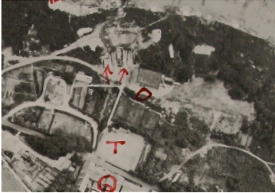
Figure 5 Enhanced detail of the aerial plot: the scarring to the landscape to the right of the Instrument Room is the spoil removed during the tunnel excavation. This spoil was initially moved by hand, but was later transported by light railway.
