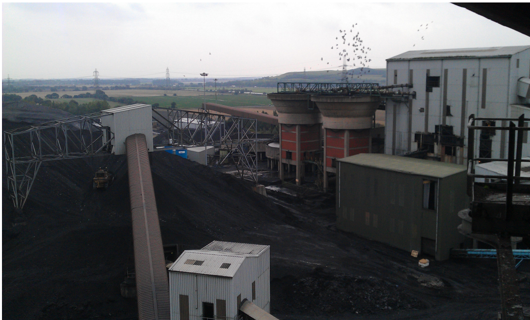
Figure 2.6: Coal Preparation Plant (UK Coal)
