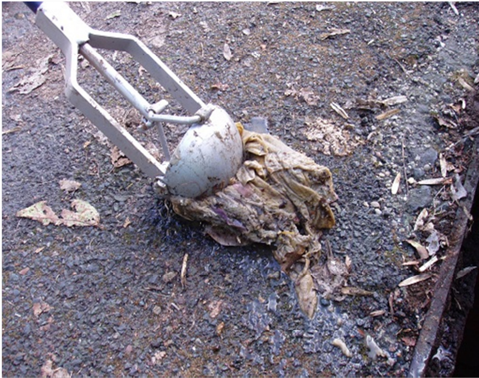
Figure 3-3 Location NIW/A - A ‘gully grab’ used to remove blockage material from the sewer
