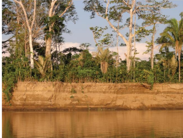
Figure 3: Typical bank sections along the study reach: a) Stable cutbank consisting of clay-rich material at Bend 72; b) Bank composed of silty, highly erodible sediments, with evidence of vertical layering.
