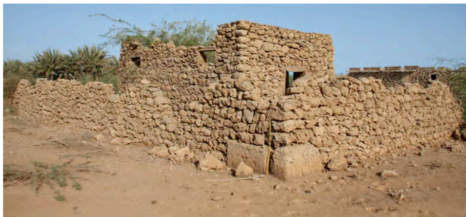
Figure 3: Ashlar blocks re-used at al-Buq'a.
