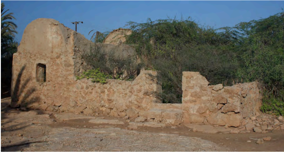
Figure 23: Abandoned mosque with barrel-vaulted roof at al-Qusar.
