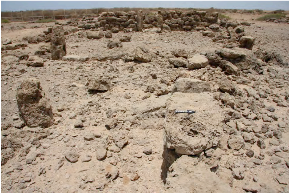
Figure 14: General view of the buildings at Wadi Matar Jīm.
