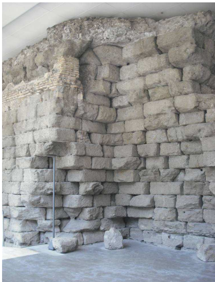
Fig. 4.33 Cappellaccio tufa blocks of the temple of Jupiter Capitolinus substructures with concrete visible on top.
