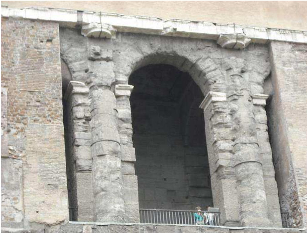
Fig. 4.28 Travertine (white elements) used for the architrave and capitals of the 'Tabularium' arcade.
