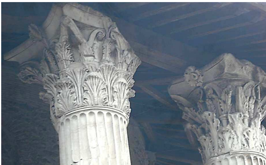
Fig. 3.8 Original capital on the left, replacement on the right. Note the different symbols (wheat and snake) in the flower, as well as the difference in leaves and use of drilling on the replacement.
