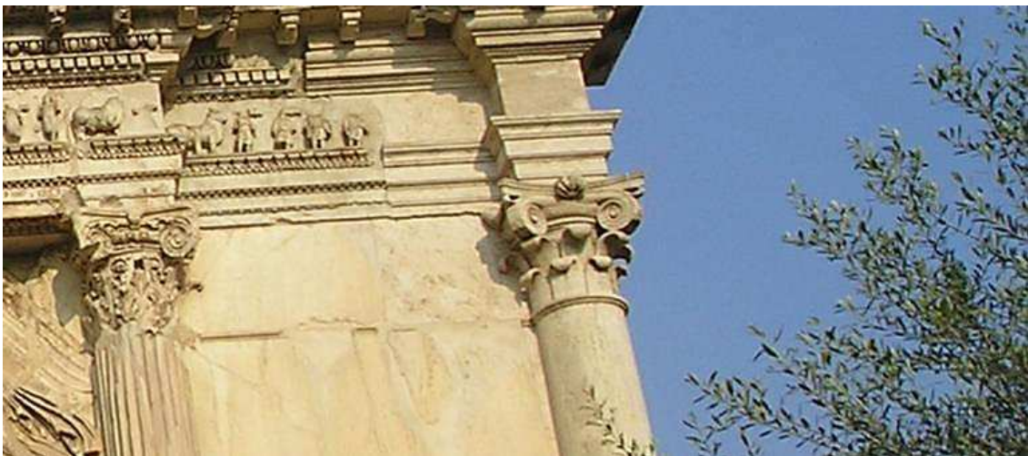
Fig. 3.10b Detail showing the deliberate absence of detailing on the restored elements of the arch.
