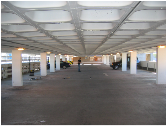
445 Figure 16: R-P car park, waffle-slab; the mode shape engages the majority of the car park level, 446 whose structural form is the same as the upper level.
