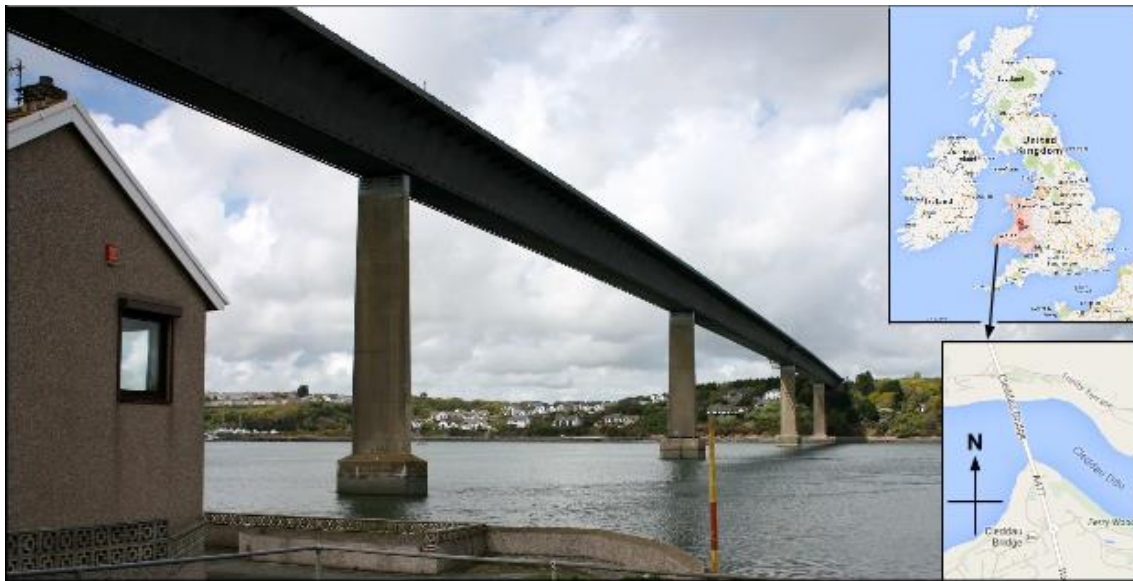
Figure 1. The Cleddau bridge (looking from east of Pembroke dock) (left) and its geographical location (right). (Courtesy: Pembrokeshire County Council)
