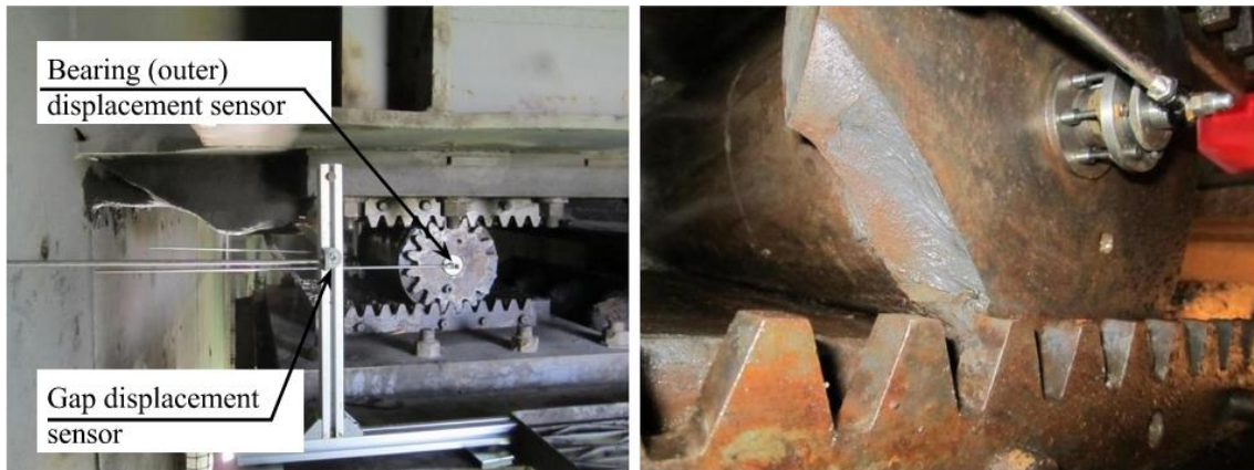
Figure 7. Instrumentation for measuring east bearing and east gap displacements (left) and sensor connection to a bearing (right). (Courtesy: Pembrokeshire County Council)
