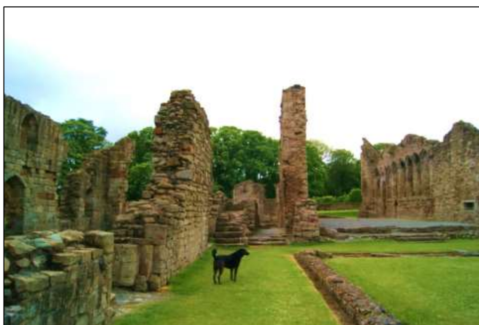
Figure 48: View of Basingwerk Abbey to the east (photo by the author).
