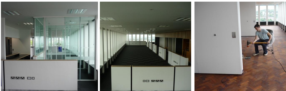
Figure 3: Half-demolished masonry partitions, cleared floor and lightweight steel frames for new fixed partitions.
