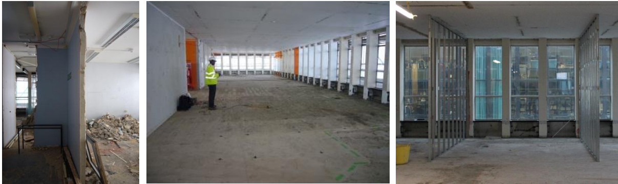
Figure 3: Half-demolished masonry partitions, cleared floor and lightweight steel frames for new fixed partitions.
