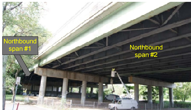
Figure 3. Picture of spans #1 and #2 (view from the eastside of the bridge)
