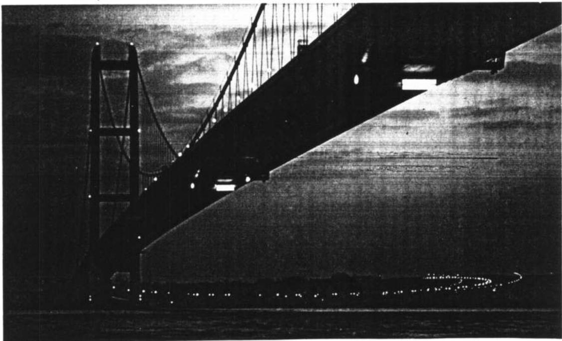
Fig. 6b Service gantries carrying horizontal, vertical optometer targets at quarter, mid span and vision system target at midspan
