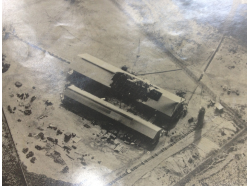
Fig 9 Aerial photograph of fire-damaged transmitter building at MERS Perim Island, 1965 (National Archives/NA/FO953/2230)
