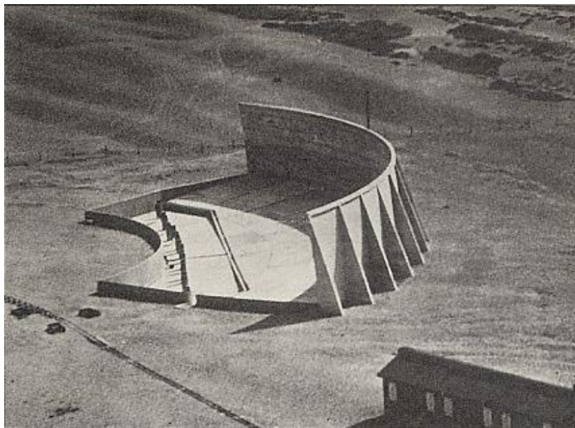
Fig.44 Aerial Photograph of Denge sound mirror, Kent. Photo: Lawrence Mayes
