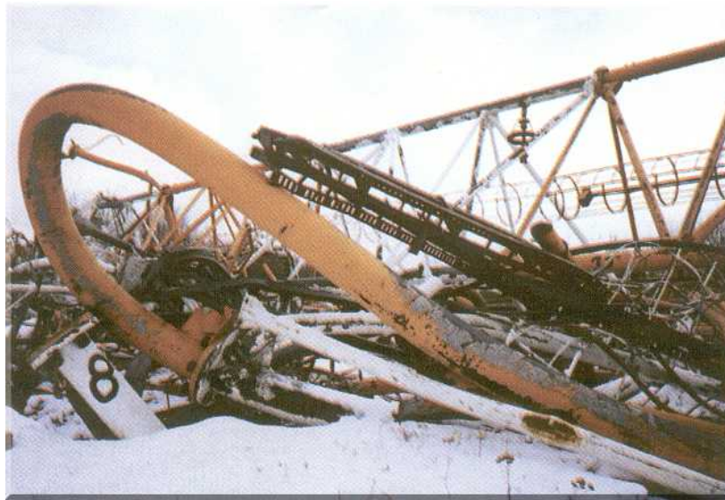
Fig. 40 Remains of Warsaw radio mast, (Present-at-hand) (Creative Commons)
