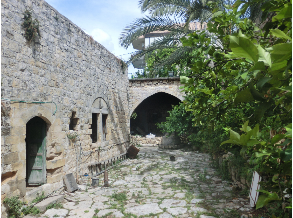
Figure 1. The courtyard of the zāwiya in Tarshiha. The door on the left leads to the main kitchen which occupies the entire building on that side of the courtyard. The space underneath the arch in the back was the summer kitchen. Photo by author, 15-05-2013.
