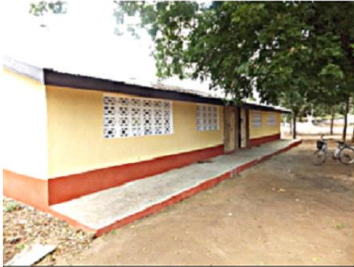
Figure 1: School building designed with screen wall concrete blocks in place of windows (Source: International Help of Missions)
