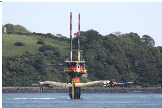
SeaGen tidal energy converter, installed at Strangford Lough in Northern Ireland. Source: https://commons.wikimedia.org/wiki/File:SeaGen,_Strangford,_June_2011_(02).JPG
