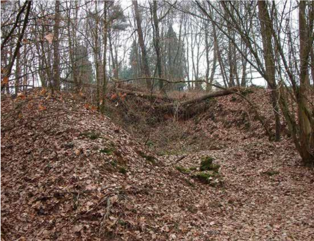
Figure 7. Example of Type IV (rations) bunker in Lager Viktor II (Manoir du Lys). Photo taken from forest track at bunker entrance.
