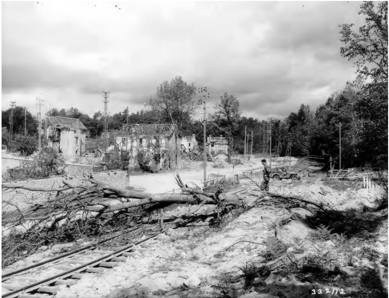
Figure 8. Photograph showing bomb damage to railway lines at Bagnoles-de-l'Orne, most probably during raids of 22 or 24 June 1944. The presence of American troops indicates the image was taken sometime after 14 August (Source: NARA 593448).
