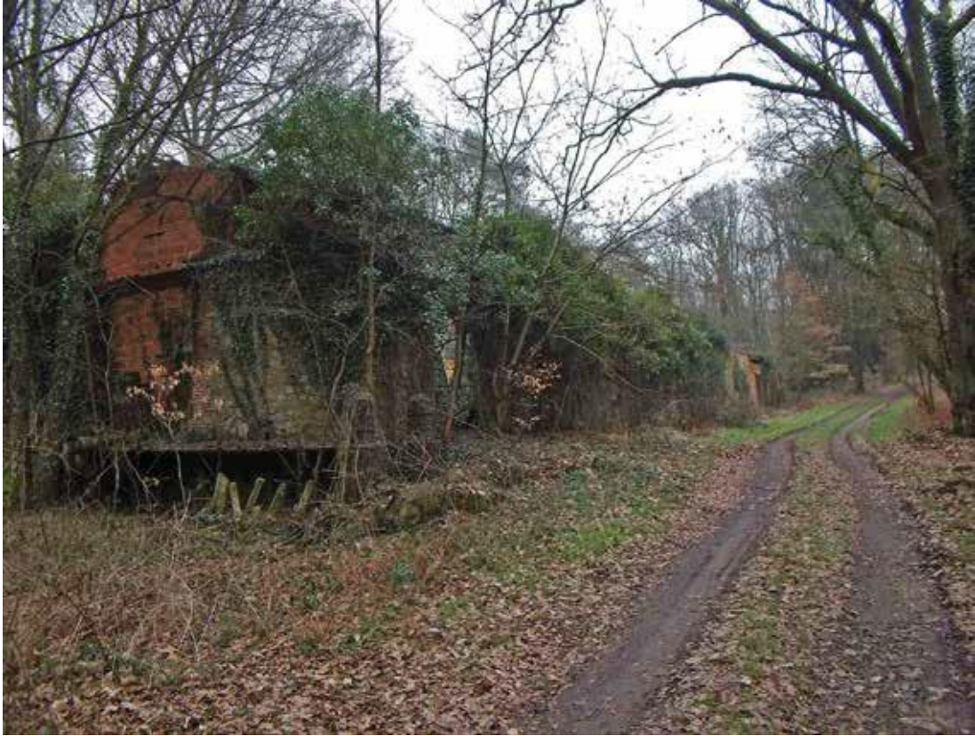
Figure 18. Derelict building at Viktor (II) near Manoir du Lys, Forêt Domaniale des Andaines, formerly used as a butchery.
