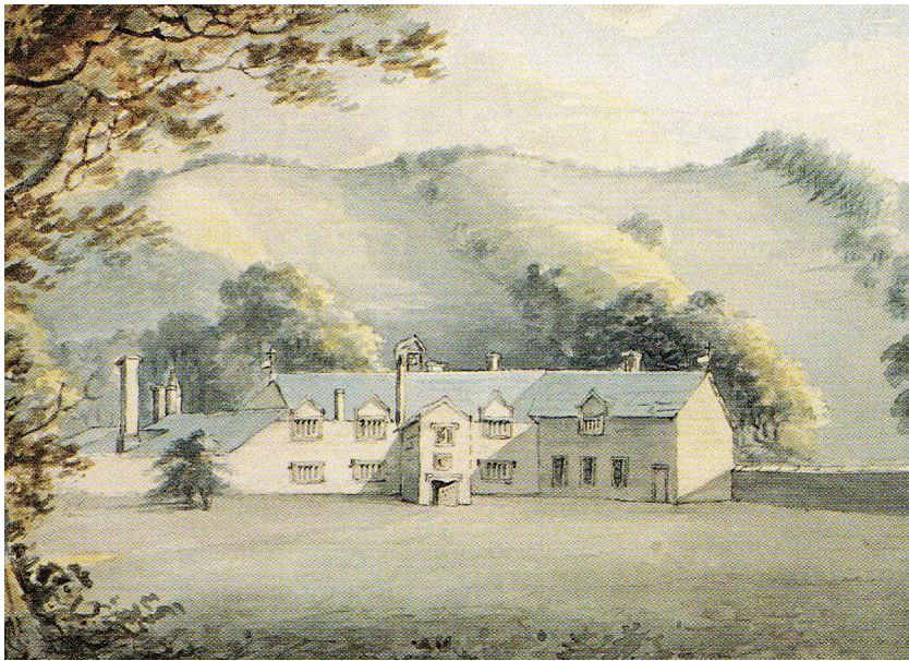
Fig.6.5: The original Oxton House that Swete demolished (Swete 1792, Journal vol. 2, opp.2).
