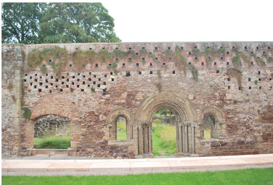
Fig.6.16: The horizontal top of the wall that Swete left out and he made the windows into arches (2015 Source: author).
