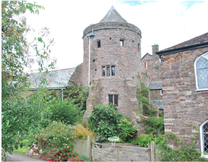
Fig.2.4: The south tower of Tiverton Castle with a pointed roof and new buildings to the west (Source: author).
