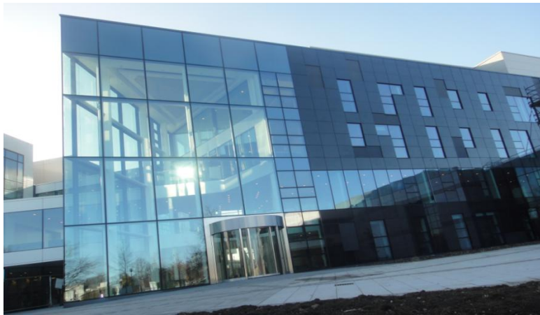
Fig. 1 Completed Charles Institute Building
