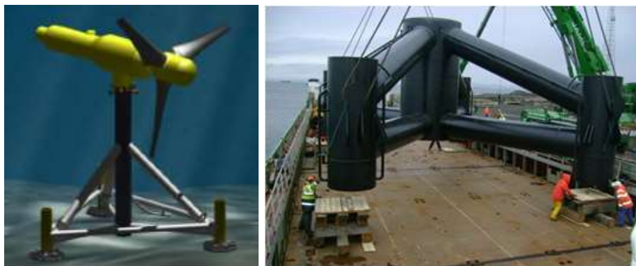
Figure 14: Pin pile foundation configurations ( left ) Alstom/TGL 1MW turbine (image source: [38]) and ( right ) Lifting of the MCT SeaGen quadrapod foundation
