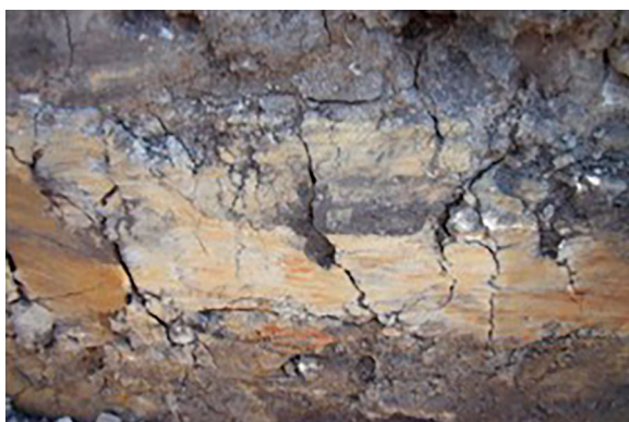
Figure 4.0 Illustrates the surface cracking evident on the grave walls.
