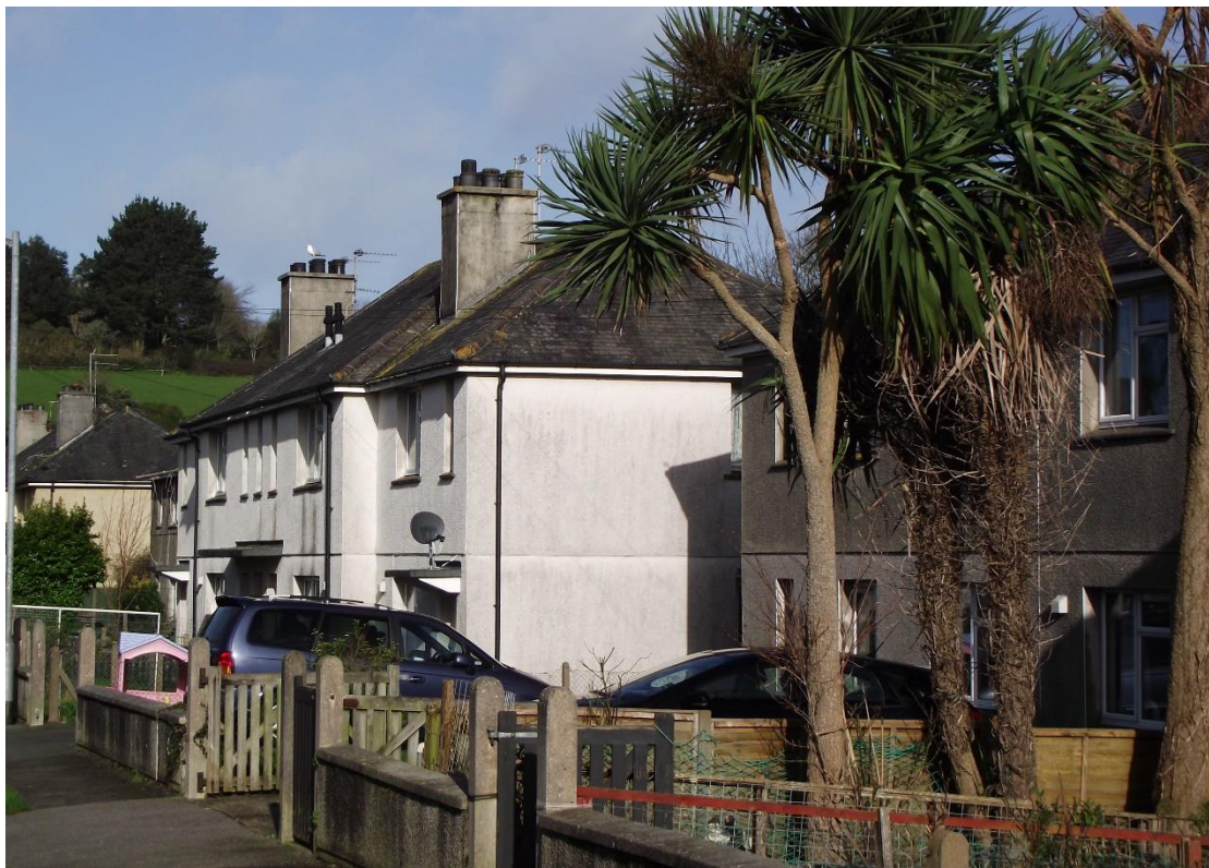
Figure 8.2: Terraced Housing on Treneere.
