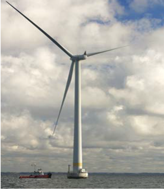
Fig. 2. The picture shows a Siemens SWT-2.3-93 in Lillgrund [40].
