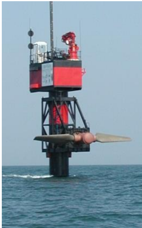
Figure 2-7: 300kW MCT Seaflow installed in 2003 off Lynmouth, Devon. Image copyright of Marine Current Turbines Ltd, sourced: www.british-hydro.org .
