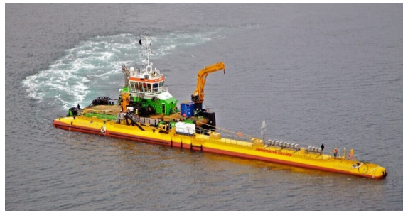
Figure 2.10. ScotRenewables Tidal Turbine (SRTT) installation ( www.greenmarineuk.com )
