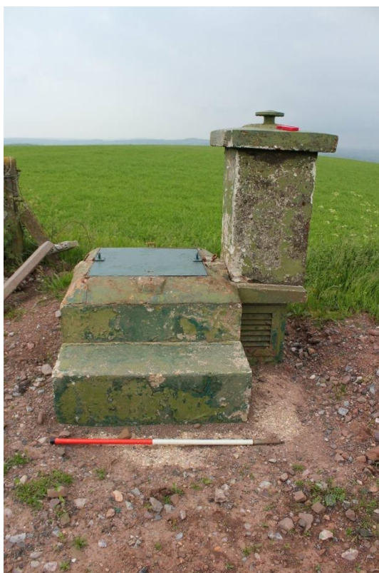
Fig.7-28. D-3, Bampton, Devon. When compared with (fig.7-25 and 7-26) the move back to order is clear. The reconstruction of the Ground Zero Indicator and refurbished entrance hatch are both markers of a covertly curated post. (source: Bob Clarke 12/06/2012)
