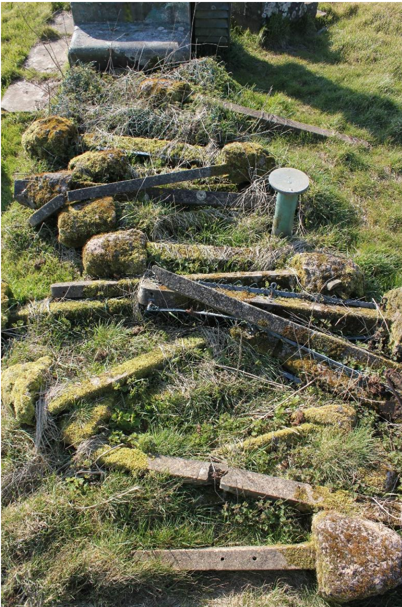
Fig.4-20. D-27, Modbury underground monitoring post. Devon The debris created by removal of the ROC post compound has been dumped on the post itself (note fixed survey meter at centre-right of picture) (Source: Bob Clarke 02/04/13)
