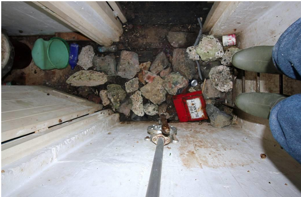
Fig.8-6. W-3 Amesbury, Wiltshire. Debris dropped from the entrance hatch above mixed with items of material culture from the operation of the underground monitoring post. The fire blanket and green bucket were both standard issue to the ROC, the drinks can, water bottle and small tin of paint are not and have been introduced from outside the secret domain. (Source: Bob Clarke 27/07/2016)
