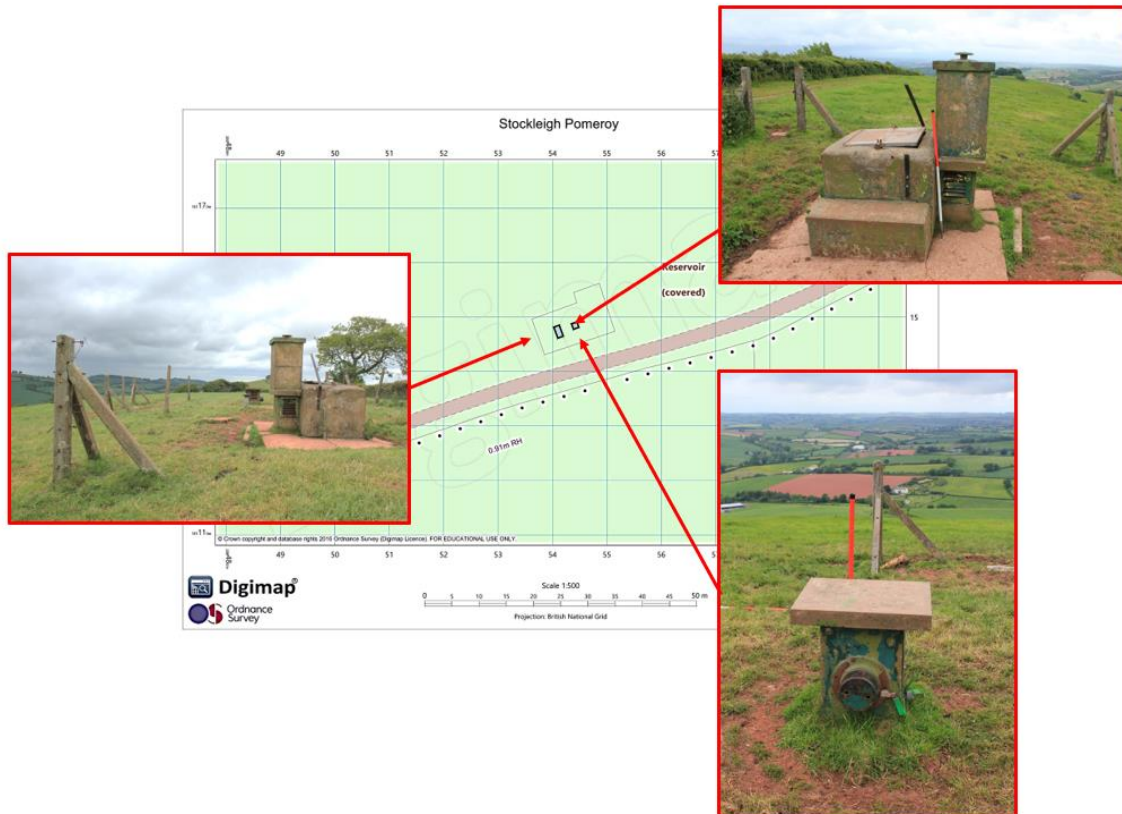
(D-41) Stockleigh Pomeroy, Devon. Location of structures. Scale: 1;500. (Left) Entrance stack with vent stack beyond, not poor state of compound fencing (Top Right) entrance stack showing damage to hatch and, now broken, metal band attempting to close off the entrance. (Top Right) Vent stack showing master post fitting and pavement slab on top of stack rather than the shallow eves lid. (©Crown Copyright/database right 2014. An Ordnance Survey/EDINA supplied service)
