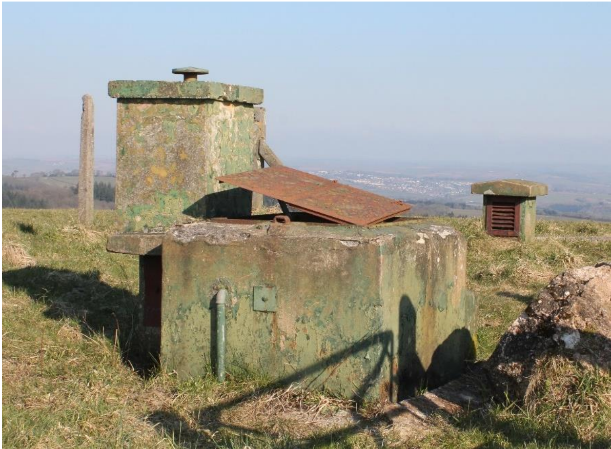
Fig.4-21. D-47 Whitestone, Devon, the entrance hatch has been forcibly opened, snapping one of the hinges. This form of interaction allows water to ingress the control room, transitioning the structure, in time, from transitional to ruined status. (Source: Bob Clarke 03/04/13)
