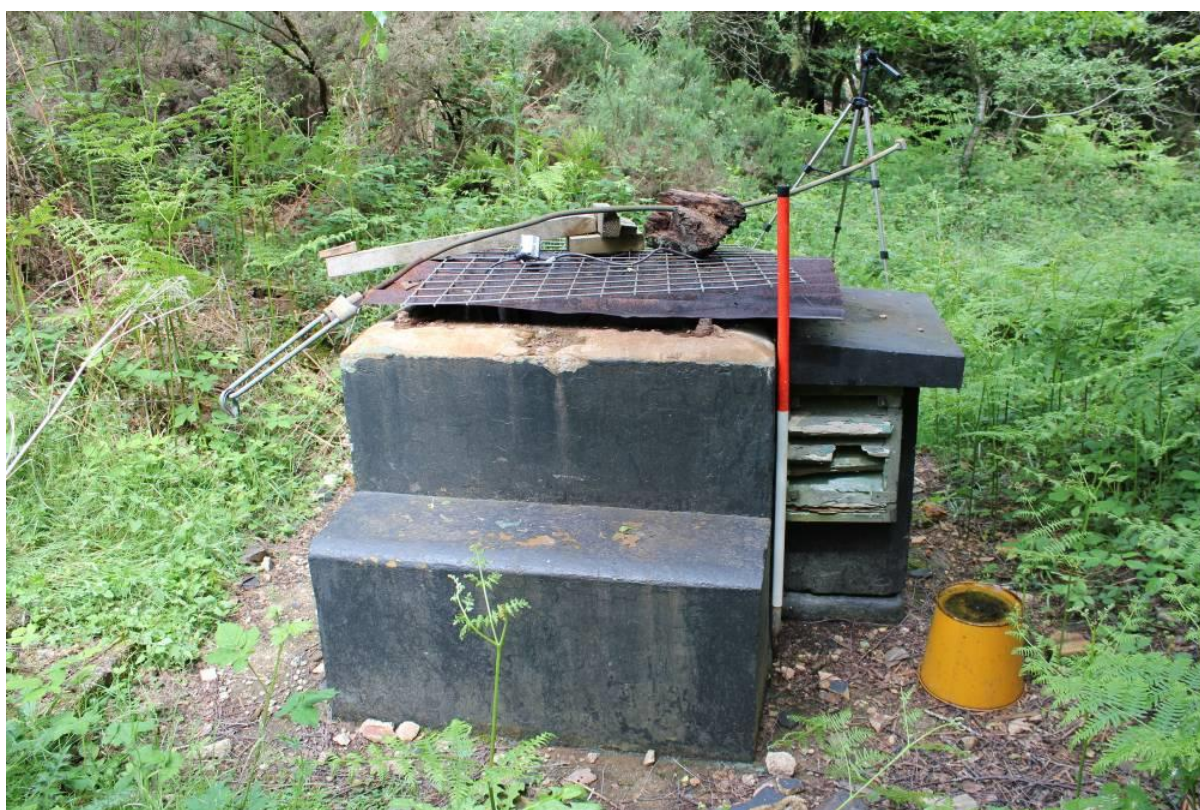
Fig.7-31. D-7, Christow, Devon. The entrance stack at Christow in the process of refurbishment. The hatch has been removed and the hole covered by a multitude of metalwork, all padlocked to the first rung of the ladder. (Source: Bob Clarke 12/06/2012)
