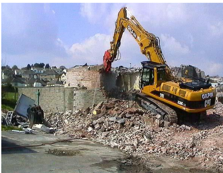
Fig.5-4. Group 11 Truro in the process of demolition in 2003. (Image courtesy of Lawrence Holmes)
