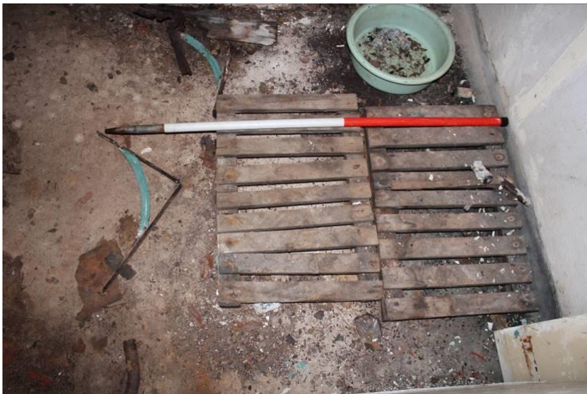
Fig.7-19. D-20, Hornscross, Devon. 'Duck boards' along with two wall mounting brackets for the equipment shelf. (Source: Bob Clarke 01/05/2011)
