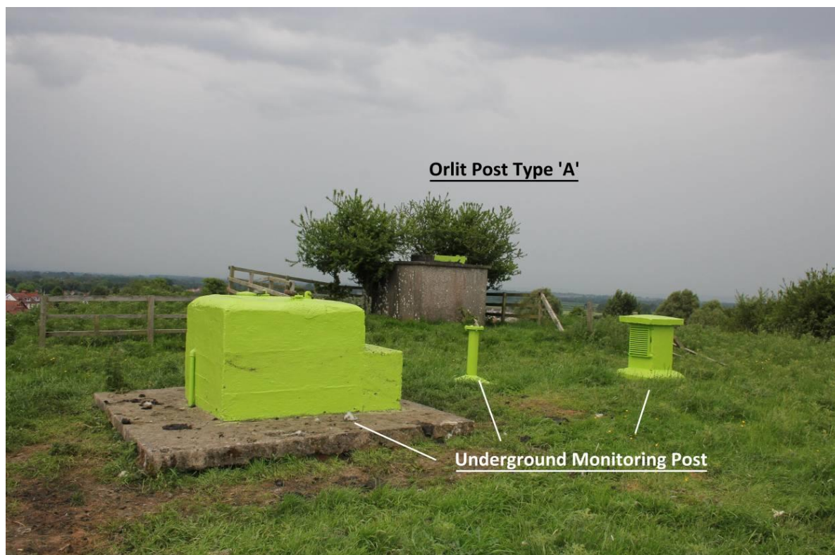
Fig.5-39. Two phases of construction at Beacon Hill, Pickering, North Yorkshire. (07/06/2014 Bob Clarke)
