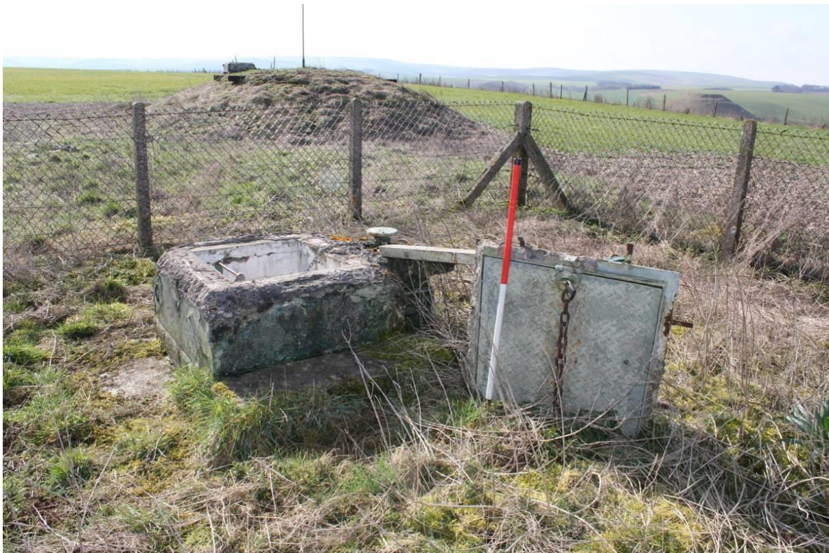
Fig.7-10. W-3, Avebury, Wiltshire. The whole hatch structure has been detached from the entrance stack. The control room below now fills with water. Beyond the compound fence is a reservoir mound, to the top right is Silbury Hill. (11/03/2012 Bob Clarke)
