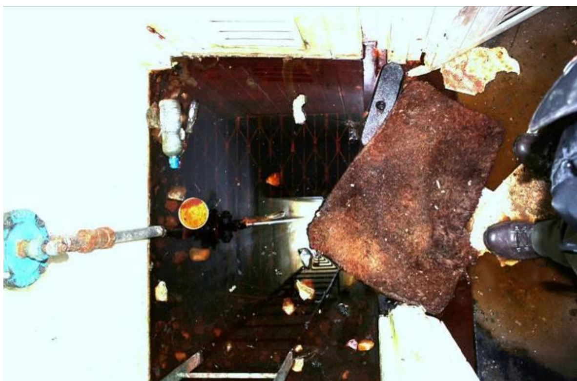
Fig.7-11. W-3, Avebury, Wiltshire. A view looking down the entrance shaft. Water ingress in the sump area of the entrance stack. The black is stagnant water. (Source: Bob Clarke 11/03/2012)
