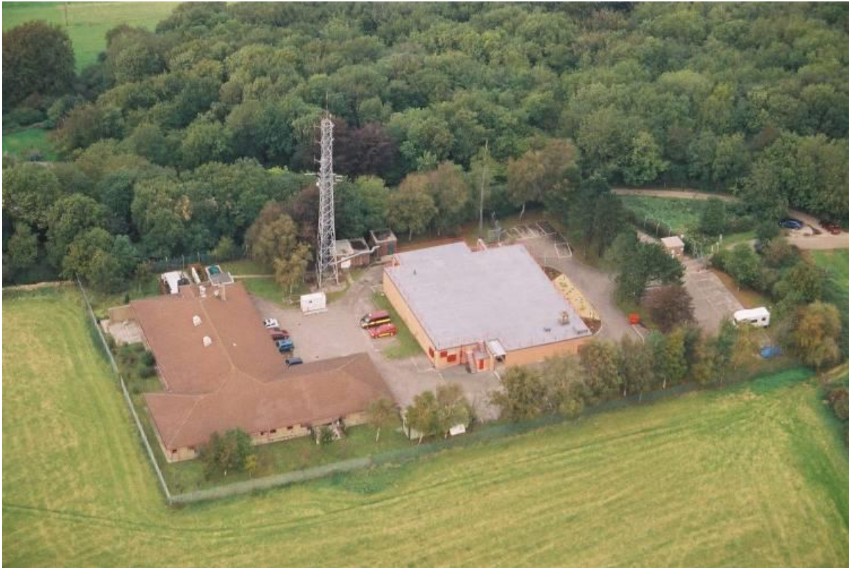
Fig.5-6. Lansdown, Avon. Southern Area UKWMO Headquarters and ROC 12 Group Headquarters looking north. The original AAOR is central to the image with the grey roof. The later UKWMO offices are to the left of the image. (Source: Bob Clarke 12/06/2006)
