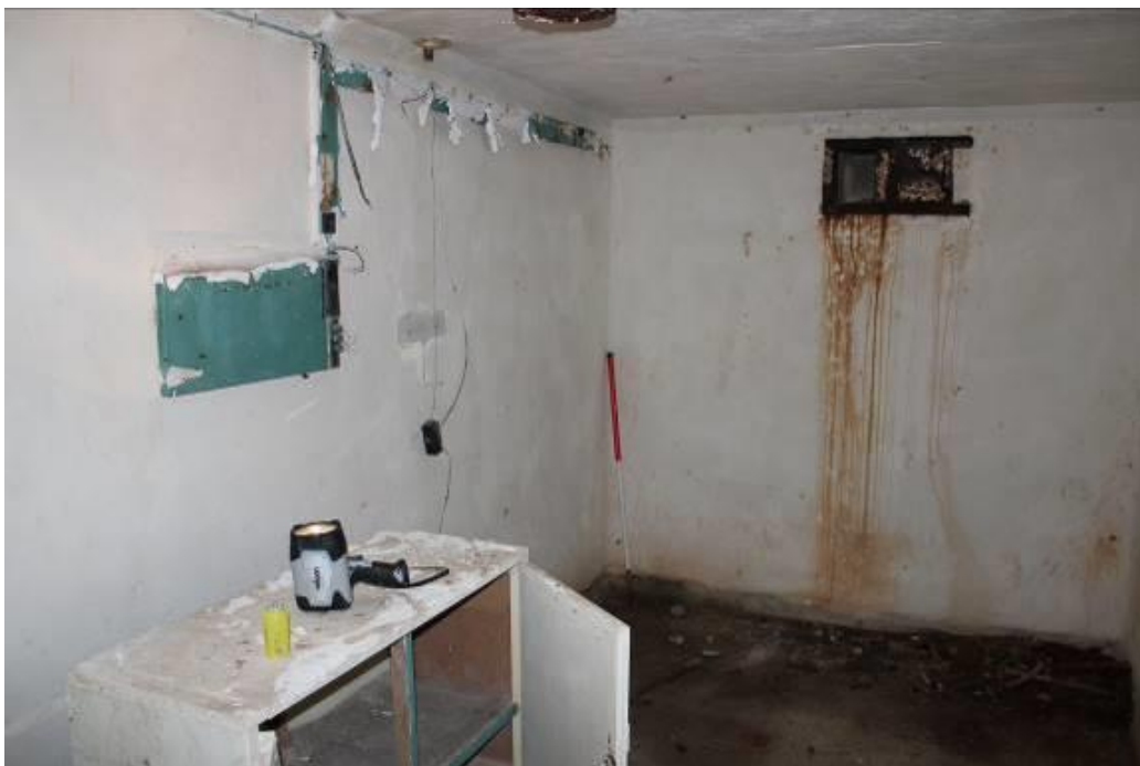
Fig.7-18. D-20, Hornsross, Devon. The control room exhibits the effects of damp. Note the deterioration around the vent (top right) caused by vegetation encouraging moisture down the shaft. (Source: Bob Clarke 01/05/2011)
