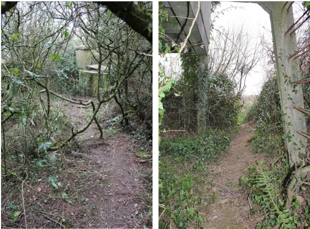
Fig.7-22 (left) looking south towards the rear of the compound and the underground element of the post. Fig.7-23 (right). Looking north towards the road, note Orlit ladder and legs. Access in both directions is restricted by vegetation. (Source: Bob Clarke 01/04/2013)
