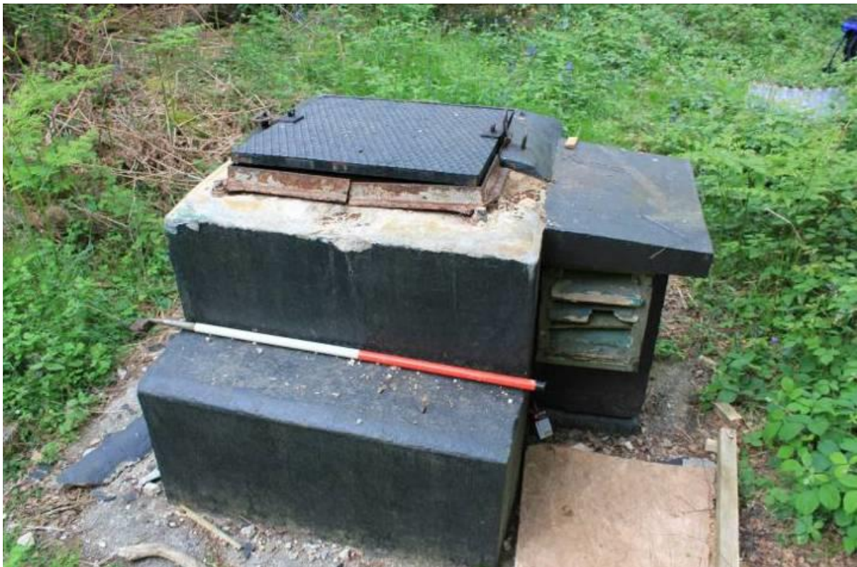
Fig.7-30. D-7, Christow, Devon. The entrance stack at Christow ROC post. Evidence is clear that a concerted effort has been made to enter the post forcibly. Note also damage to the wooden vent (Centre right) (Source: Bob Clarke 05/06/2011)
