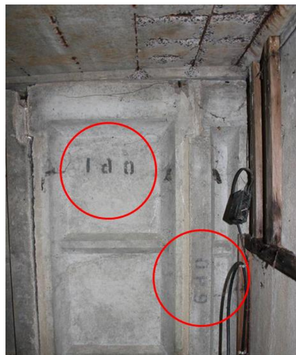
Fig.5-14. D-44 Teignmouth, Devon. Orlit Type 'B'. Floor planks bearing two distinct marks. 'F' and 'B', both capitalised and executed using a finger in the, still wet, concrete cast. (Source: Bob Clarke 10/07/2014)
