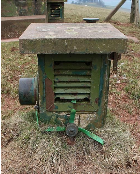
Fig 6-4. D-41 Stockleigh Pomeroy Devon, 10/D.2 opened in June 1959. The dome fitted on the left of the vent stack maintained support for a large aerial. Earthing straps are also visible in case of lightning strikes. (Source: Bob Clarke 01/04/2013)
