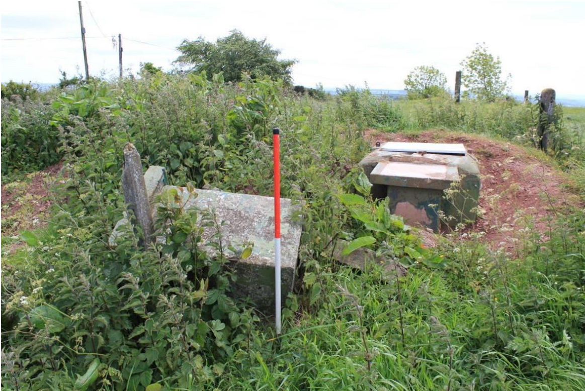
Fig.7-27. D-3, Bampton, Devon. By the time of the baseline survey for this project the process of abandonment had taken a positive turn. Soil was being removed and items of post furniture restored. (Source Bob Clarke 27/05/2011)
