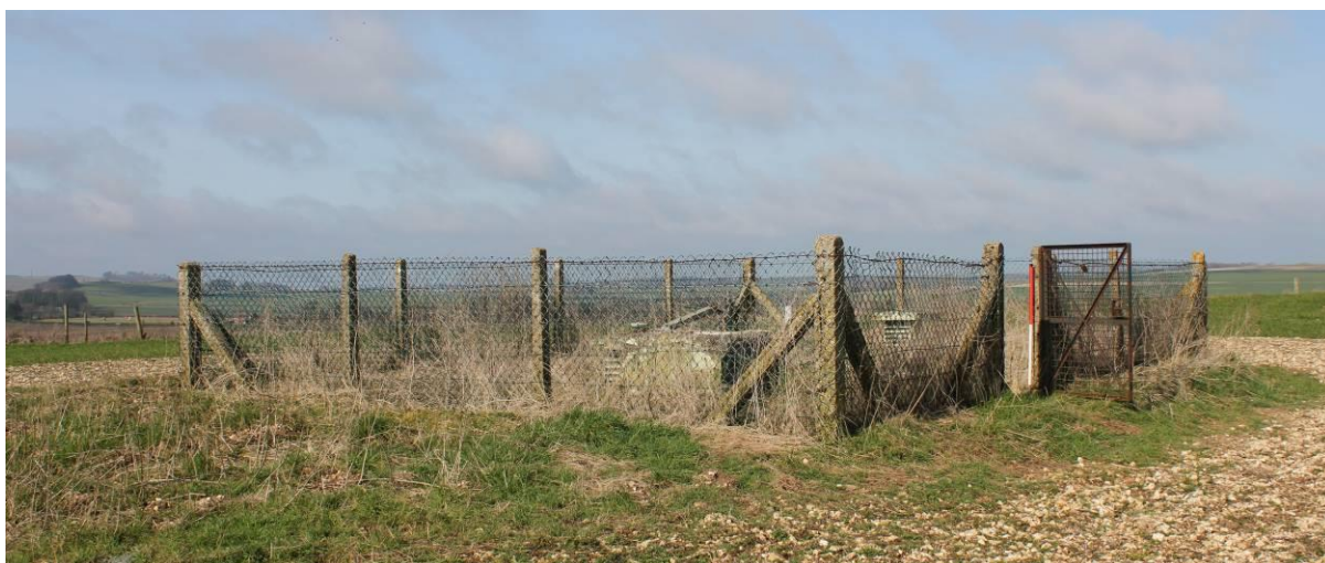
Fig. 6-3. The compound fence at Avebury Underground Monitoring Post, Wiltshire, Post14/B.1 opened in June 1961. The compound fence is intended to be stock proof. I suggest it was latterly interpreted as concealing 'deviant' activities. Range Pole 1m. (Photograph Bob Clarke 17/11/2013)
