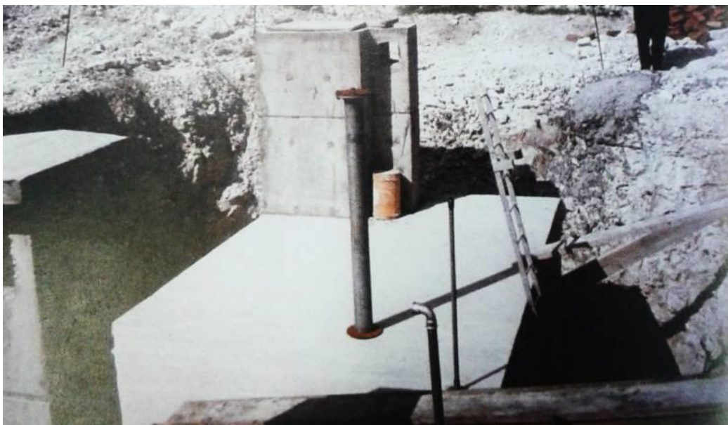
Fig.5-23. The finished structure prior to applying the pitch coat to waterproof the structure and then reburial. Note the instrument pipes attached to the roof. Unknown post. (Courtesy of The Royal Observer Museum)
