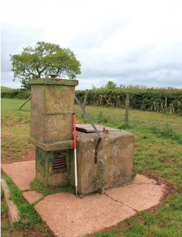
Fig.7-45. D-41, Stockleigh Pomeroy, Devon. The weather and lack of maintenance is adding to the overall degradation of the site. (Source: Bob Clarke 01/04/2013)
