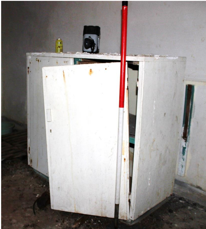
Figure. 4-23, D-20 Hornscross, Devon, Furniture and fittings, such as this cupboard, were standard issue to all underground monitoring posts. Examples of it were consistently located at nearly all posts. (Source: Bob Clarke 01/05/2011)
