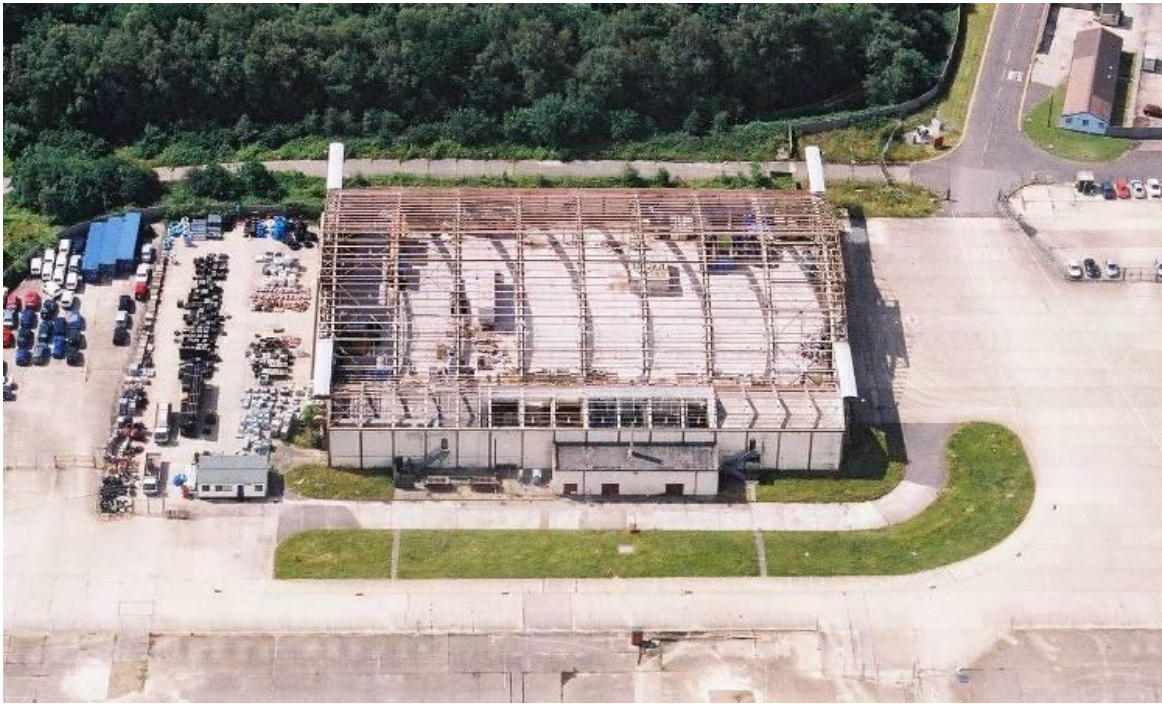
Fig.4-14. Aircraft Hangar at Greenham Common, Berks in the process of dismantling, 2004. The value of structures, especially those in the HO Operational Spaces, is often in their scrap value. Chaos through human action is compounded by meteorological conditions. (Source: Bob Clarke 02/06/2004)
