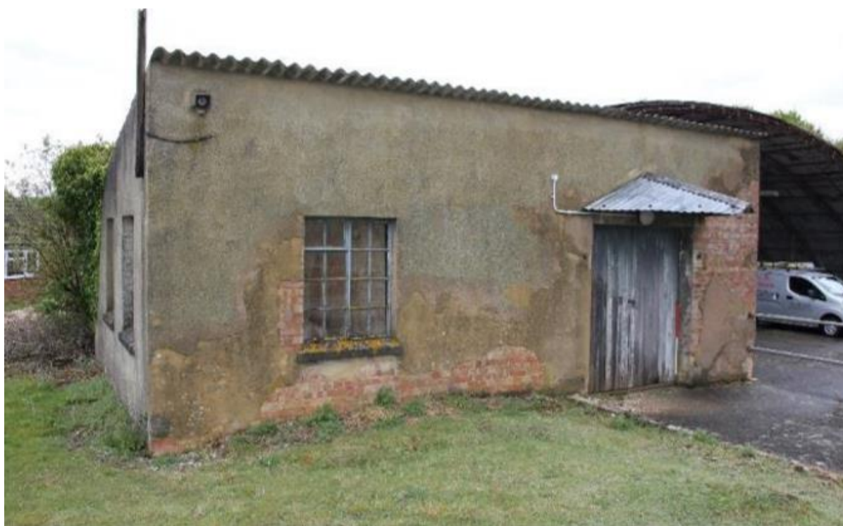
Fig.4-15 Building 310 Boscombe Down, Wiltshire. Note the poor state of the rendering around doors and windows. (IMG_0054 created 6 May 2015 ©QinetiQ Ltd - with permission)
