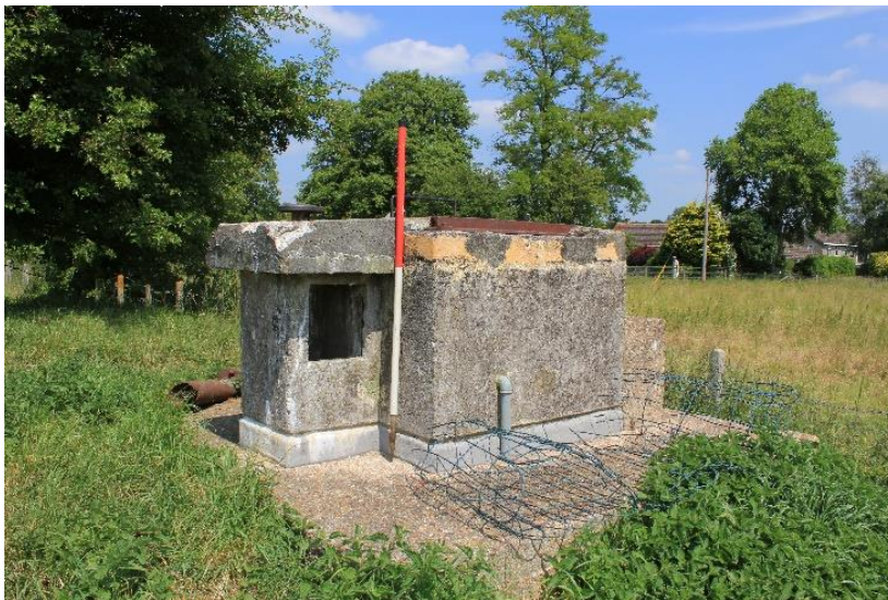
Fig.4-24. W-7, Sutton Veny, Wiltshire is a classic example of a ruined ROC Post. The post has no vent stack, or other equipment fittings and the entrance stack is devoid of grills. (Source: Bob Clarke 07/07/2013)
