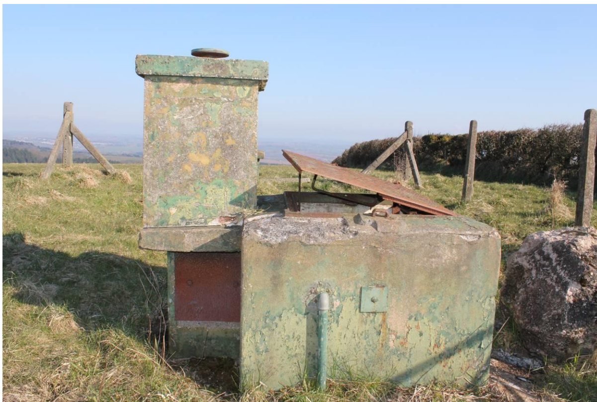
Fig.8-4. D-47 Whitestone, Devon. The hatch at this post has been damaged to such an extent it will not close beyond the point illustrated here. (Source: Bob Clarke 03/04/2013)
