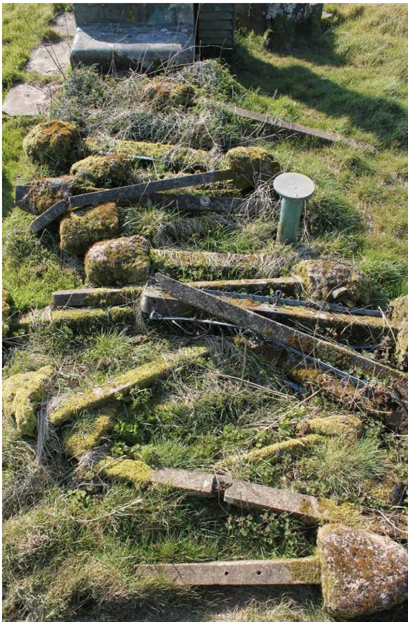
Fig.7-34. D-27, Modbury, Devon. The central area of the ROC post at Modbury is covered in the debris of the compound fencing. Ploughing also continues to erode the site. (Source: Bob Clarke 02/04/2013)
