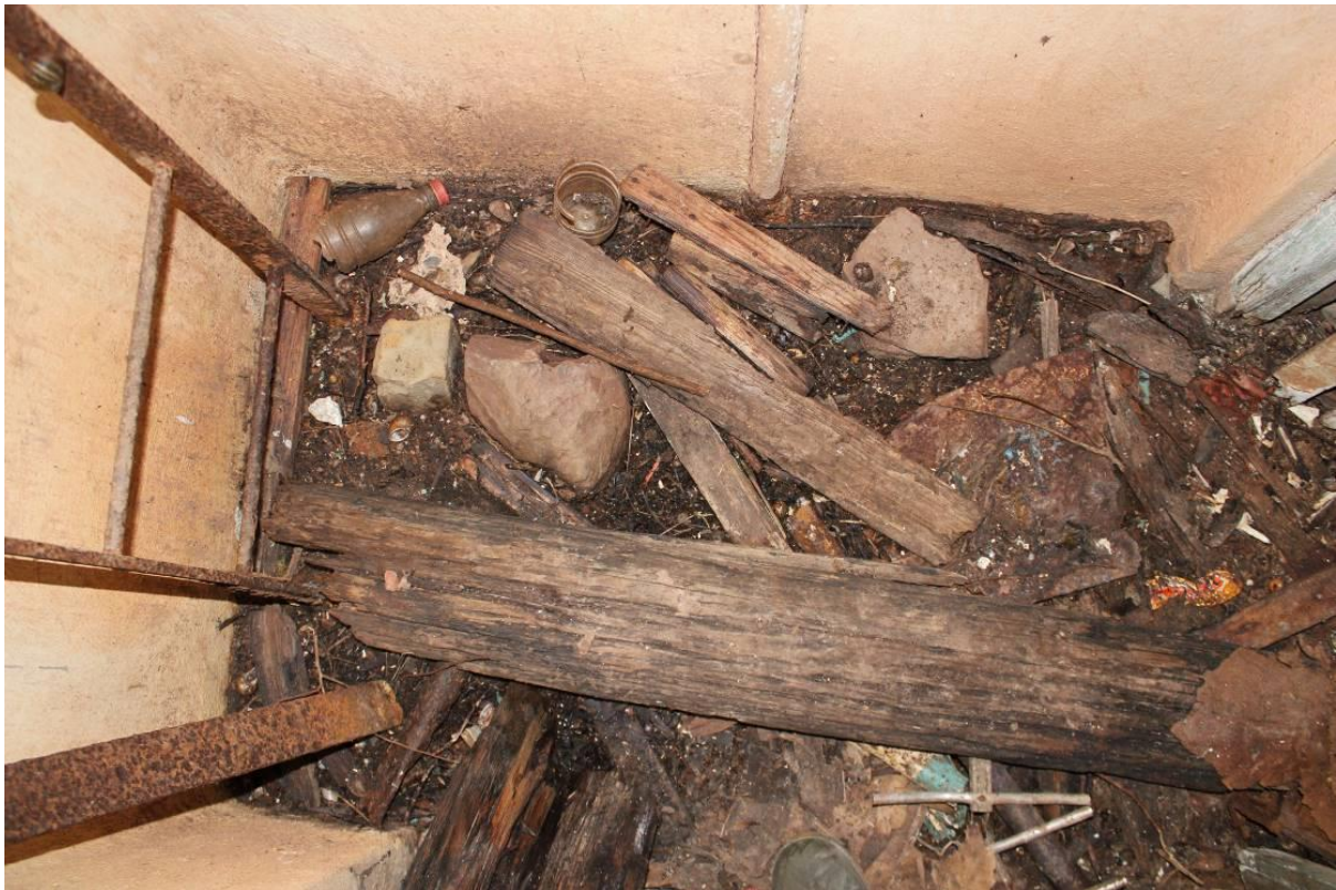
Fig.7-17. D-20, Hornscross, Devon. The sump area of the post entrance. A mixture of leaf litter and items dropped down the shaft have fouled the drainage. (Source: Bob Clarke 01/05/2011)
