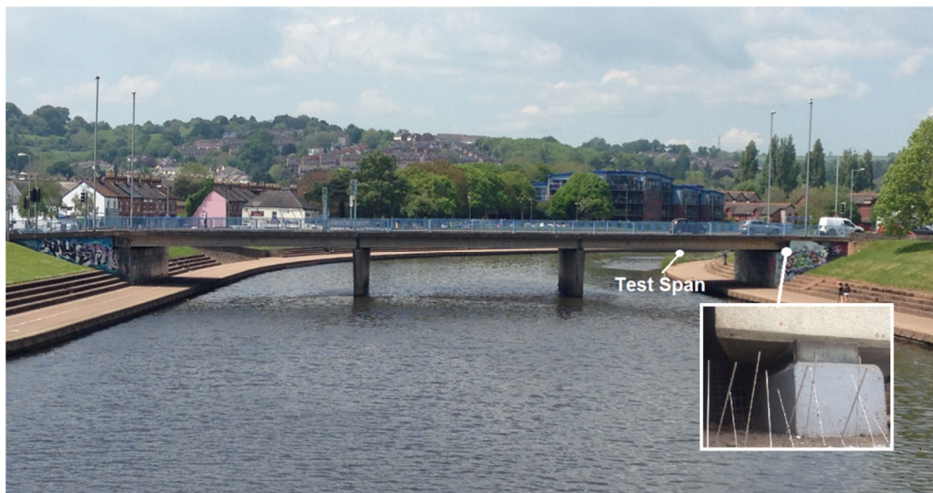
Fig. 2 Exe North Bridge spanning River Exe
