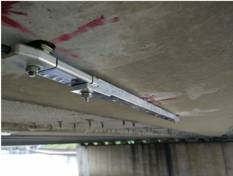
Fig. 3 Strain Transducer attached on a girder soffit with an aluminium extension rod
