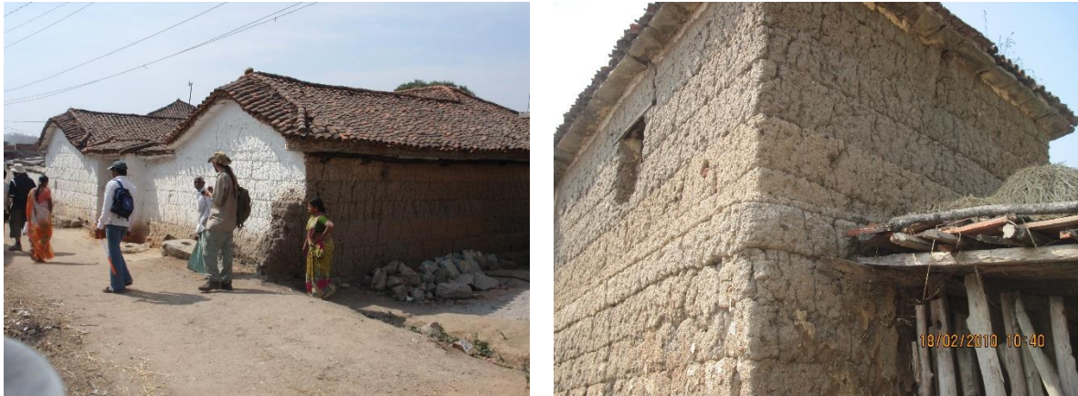
Figure 5.7 – Houses constructed of mud-courses suggesting that they must be of a considerable age.
